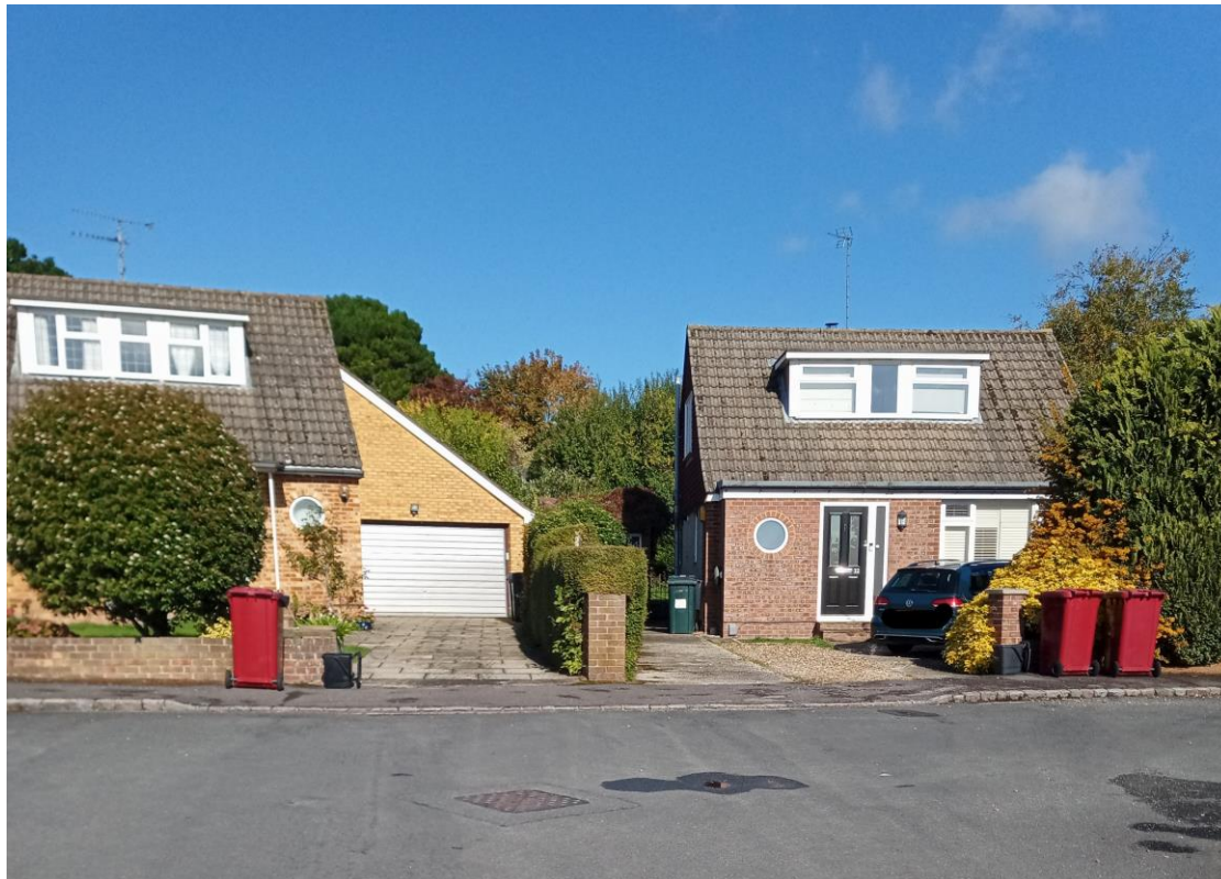
Figure 1: 22 and 24 Gurney Close frontage
