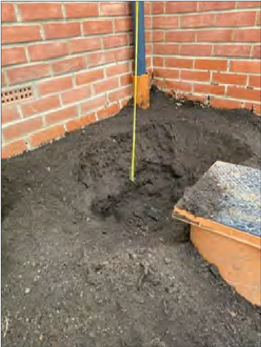
Photo 8: Confirming Clean Cover Thickness and Presence of Geotextile Break Layer within Plot 2
