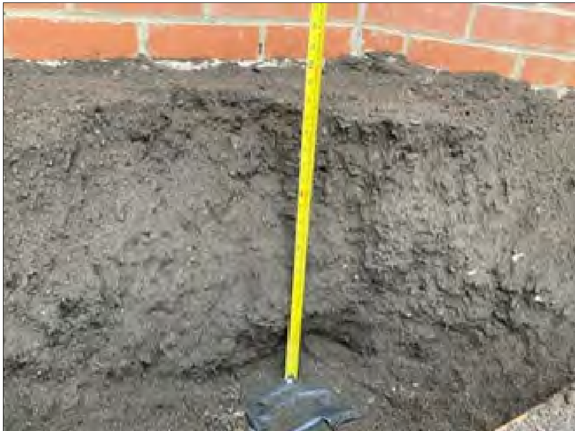
Photo 7: Confirming Clean Cover Thickness and Presence of Geotextile Break Layer within Plot 5
