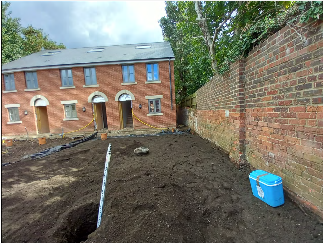
Photo 2 - Showing Location of Inspection Pit within Plot 7
