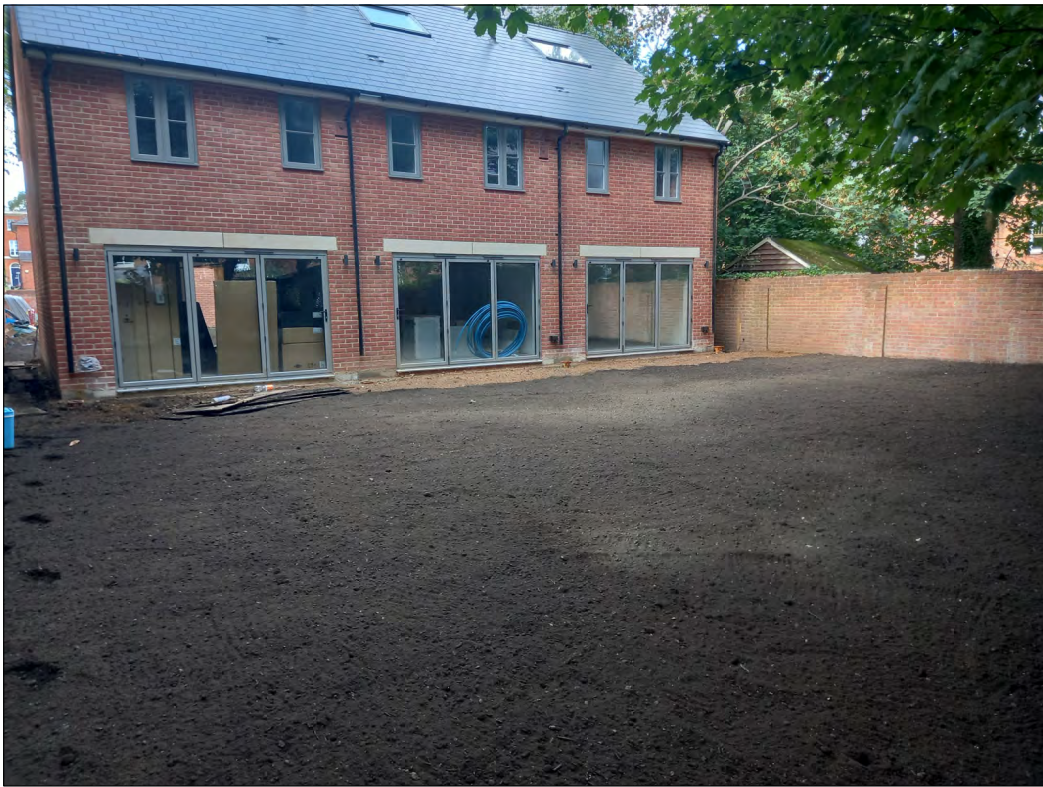
Photo 1 - Showing Completed Clean Cover within Plots 7 to 9
