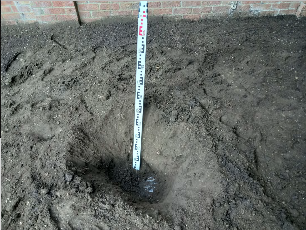
Photo 5: Confirming Clean Cover Thickness and Presence of Geotextile Break Layer within Plot 8
