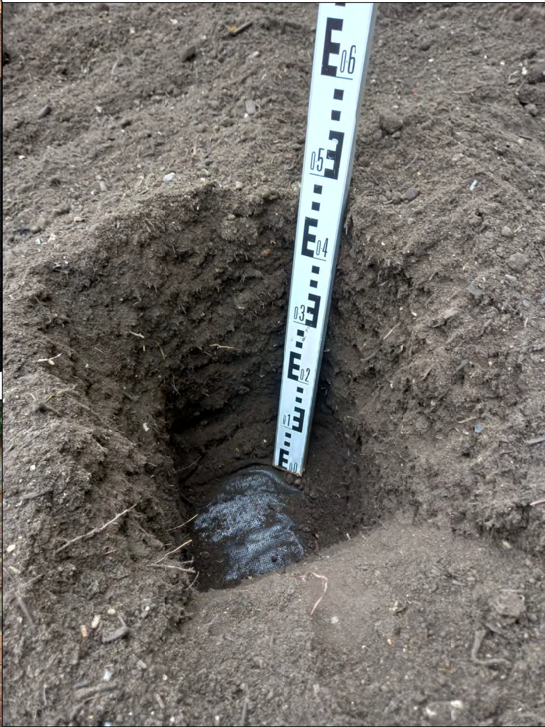
Photo 3: Confirming Clean Cover Thickness and Presence of Geotextile Break Layer within Plot 7
