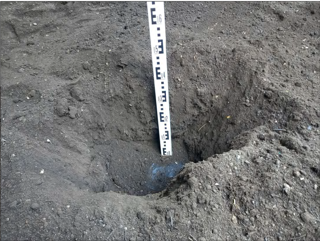
Photo 4: Confirming Clean Cover Thickness and Presence of Geotextile Break Layer within Recreational Area
