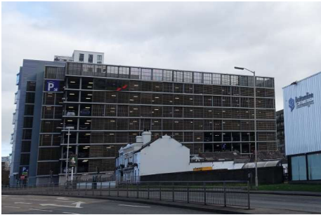
Chatham Place Multi-storey Carpark (9 Storeys)
