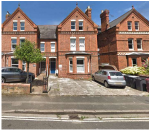
Castle Crescent: late 19th century semi-detached houses
