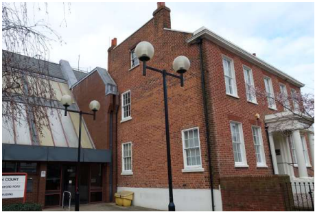
1. Mannson House - West Elevation
