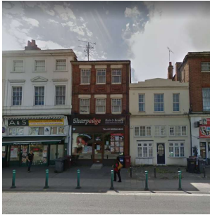
Oxford Road: retail buildings with offices or flats above
