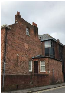
1. Mannson House - East Elevation
