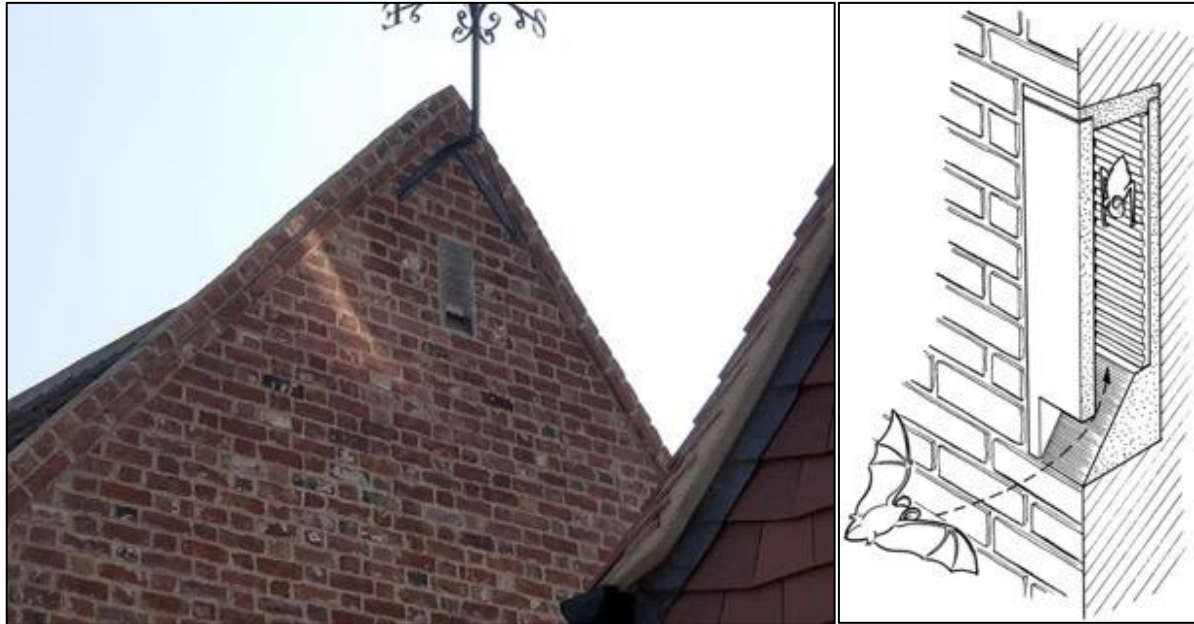
Figure 10. Left – A bat tube integrated into a brick wall. Right – a cross section diagram of a bat tube.
