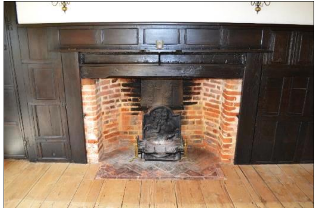
Figure 28: Exposed open timber framing, (right) detail of brick lined fireplace surrounded by the remains of 17 th century timber panelling- interestingly parts of this panelling have been re-used elsewhere within the house
