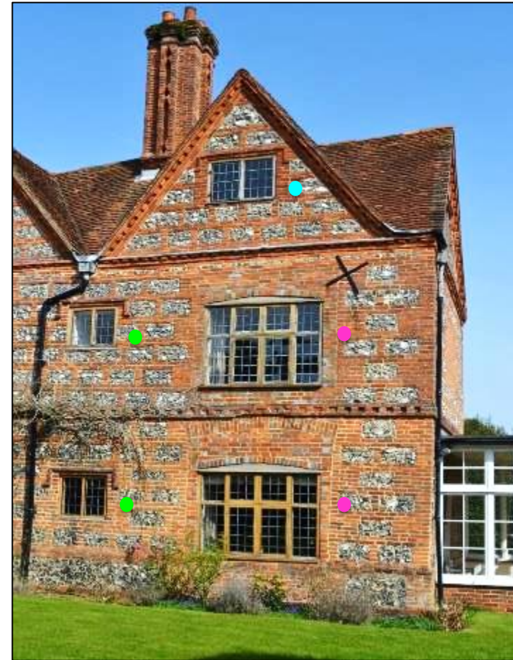
Figure 17: Details of the west elevation- (left) 20 th century porch inset with 17 th century door, (right) when compared to Figure 16 the fenestration alterations become clear, the inserted two light casement windows under hood mouldings (highlighted in green), and the 4 light mullion and transom windows which have been increased in size from the early 20 th century
