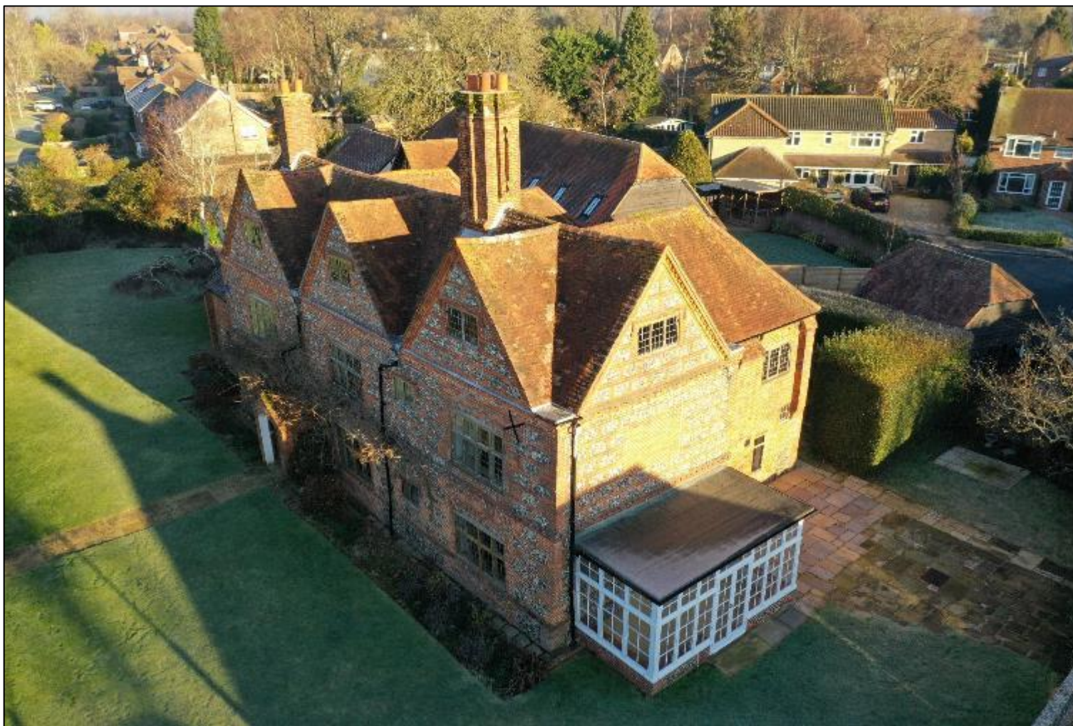
Figure 8: Drone photo overlooking the west and south elevations
