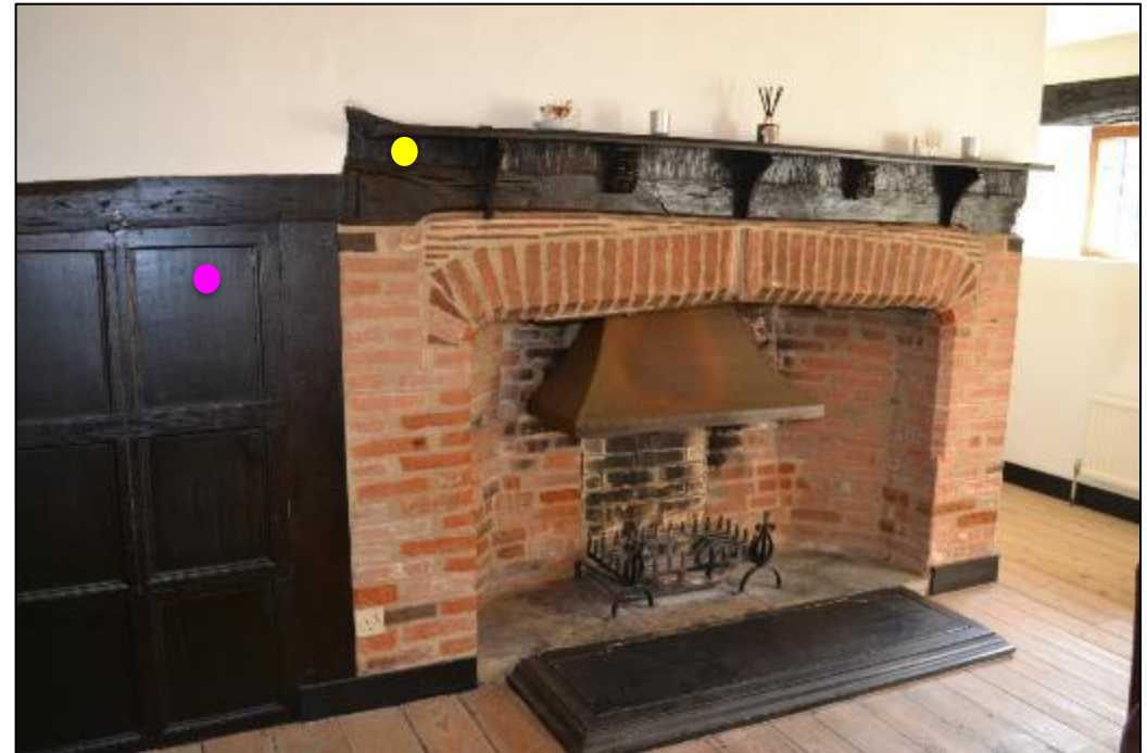
Figure 27: Exposed timber framing throughout, (right) remains of 17 th century timber panelling (highlighted in pink) and large Tudor depressed brick arch fireplace and moulded mantel with masked brackets (highlighted in yellow)
