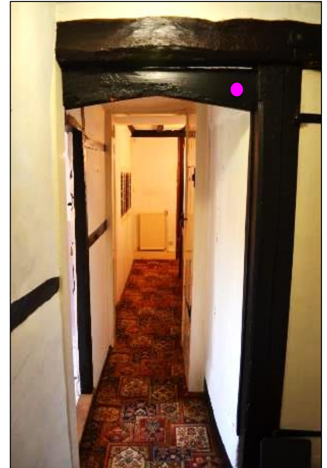
Figure 39: (left & centre) The family bathrooms located just off the main hallway, (right) interesting four centre timber arch located at the end of the hallway (highlighted in pink)
