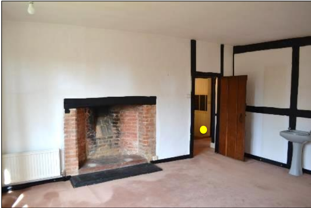
Figure 37: (left) Exposed brick lined fireplace, location of where the original stair would have emerged (highlighted in yellow), (right) internal wall of where the blocked off window on the southern elevation is located (highlighted in pink)
