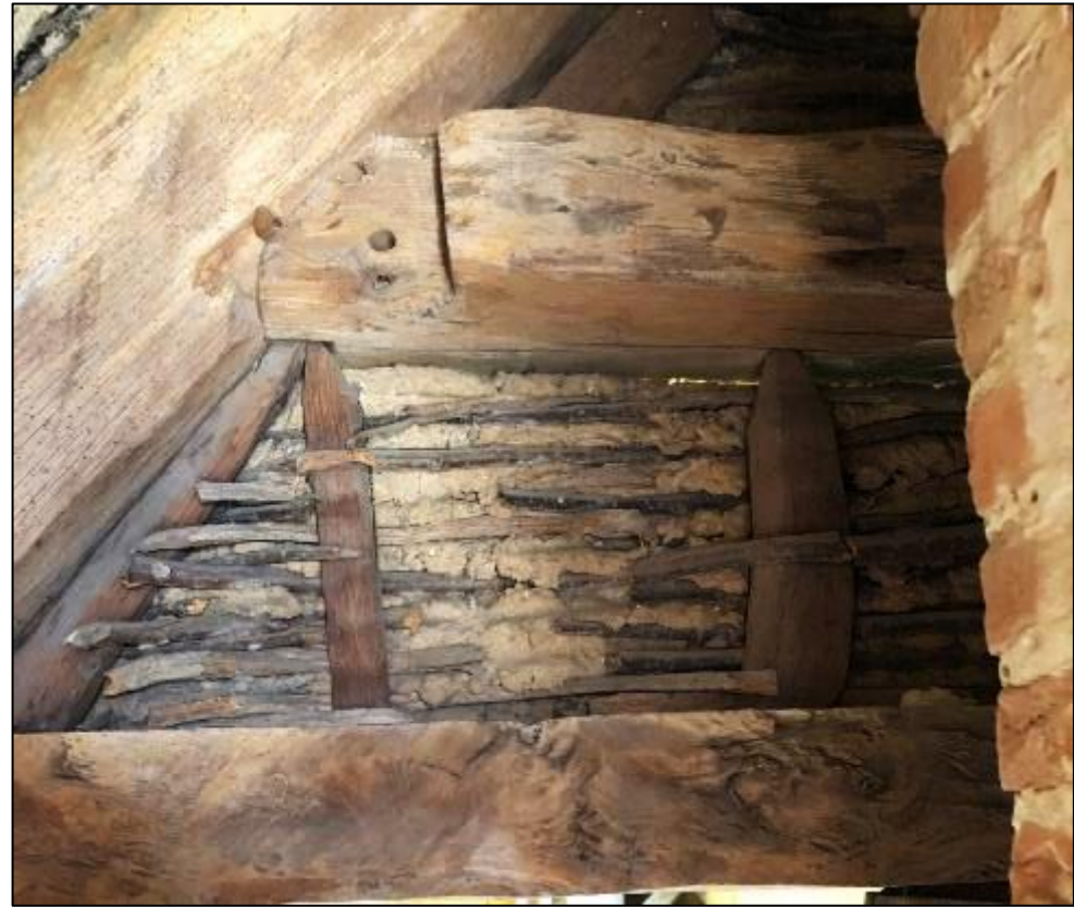
Figure 48: (left) Further examples of historic plaster panels, (right) detail of the lathes thought to be made out of willow upon which the plaster has been applied
