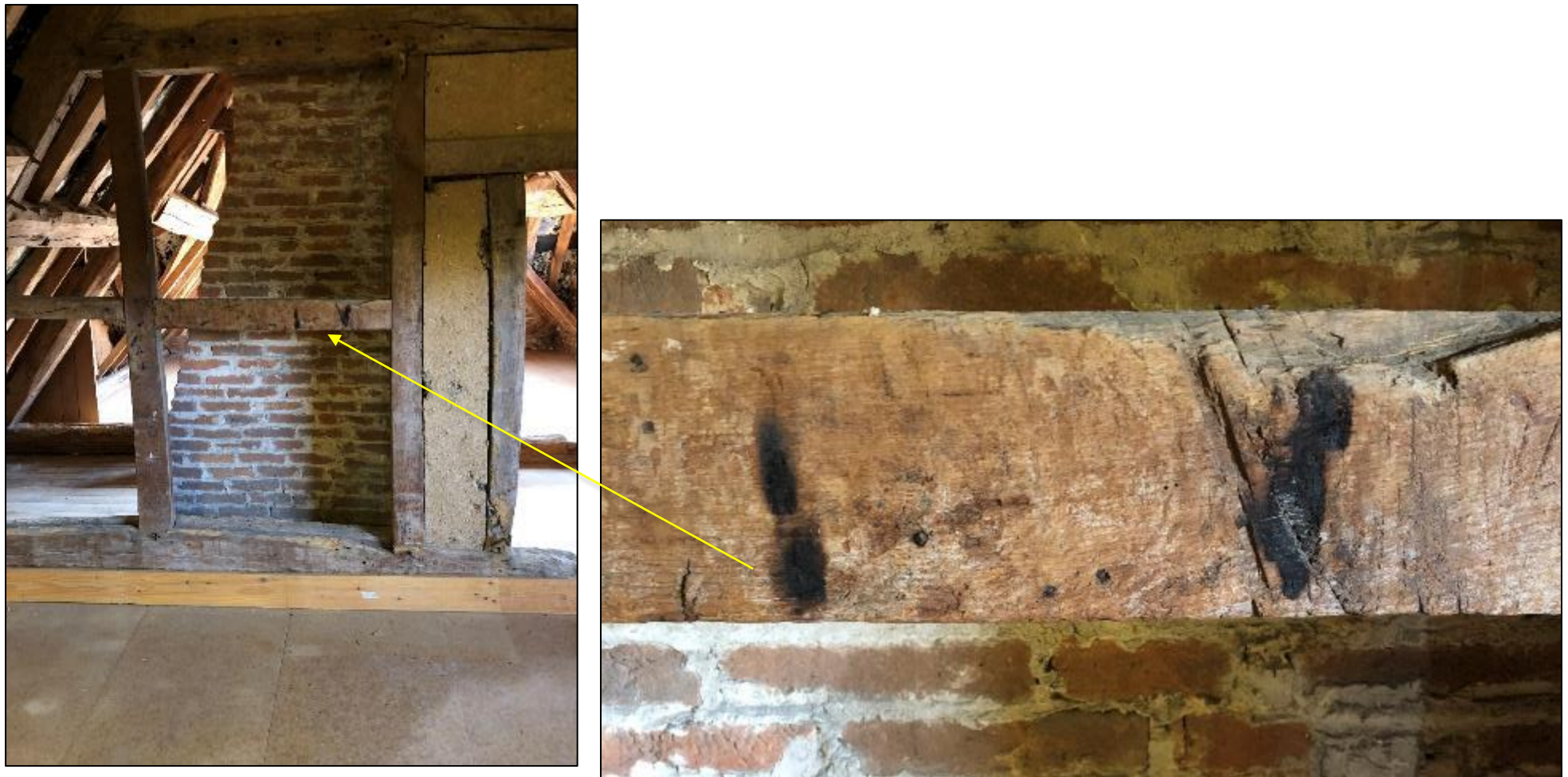
Figure 47: (left) View of timber framing and original infill around the central chimney stack, (right) example of apotropaic burn marks found throughout the attic space
