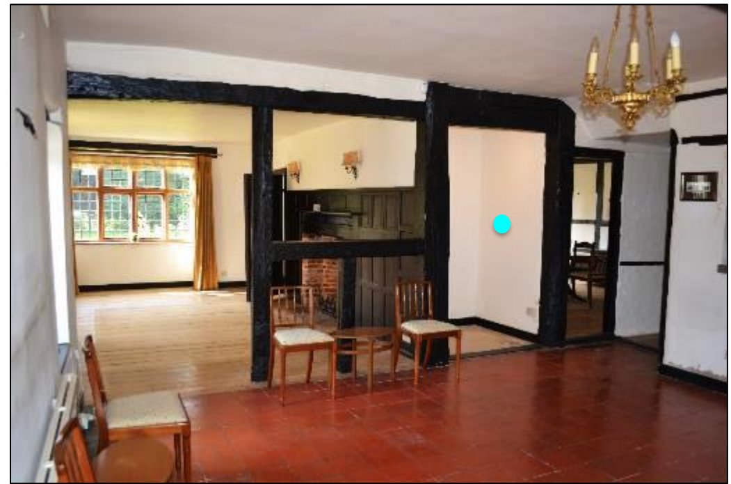
Figure 29: (left) Extended in the 19 th century (limit of extension highlighted in yellow), (right) location of former fireplace (highlighted in pink), potential location of original stair when the property was a lobby entrance plan form (highlighted in blue)
