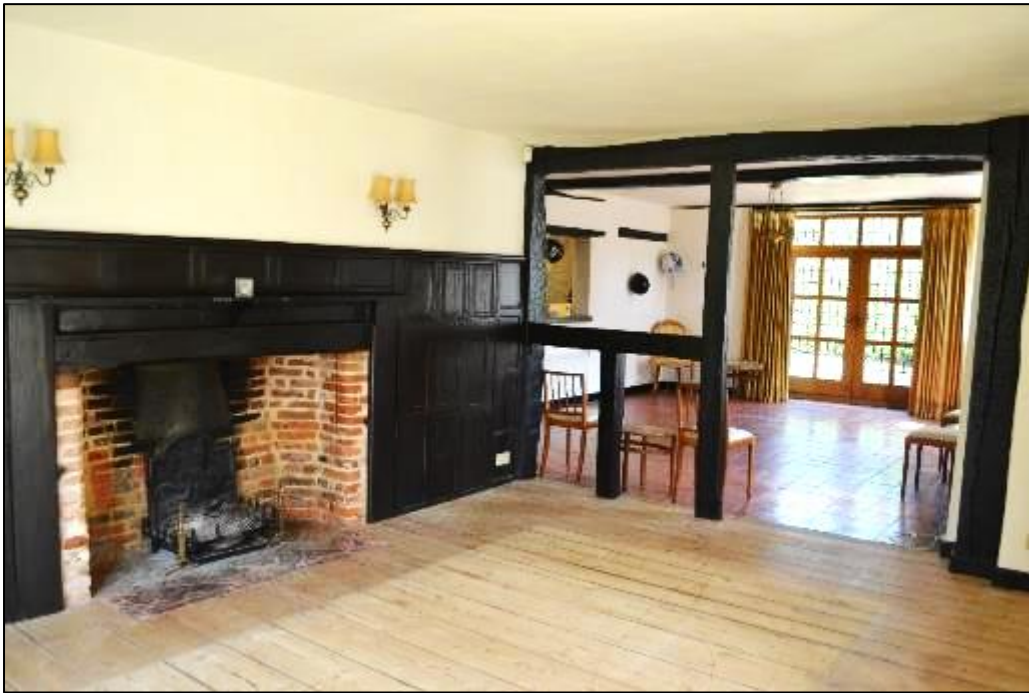
Figure 28: Exposed open timber framing, (right) detail of brick lined fireplace surrounded by the remains of 17 th century timber panelling- interestingly parts of this panelling have been re-used elsewhere within the house
