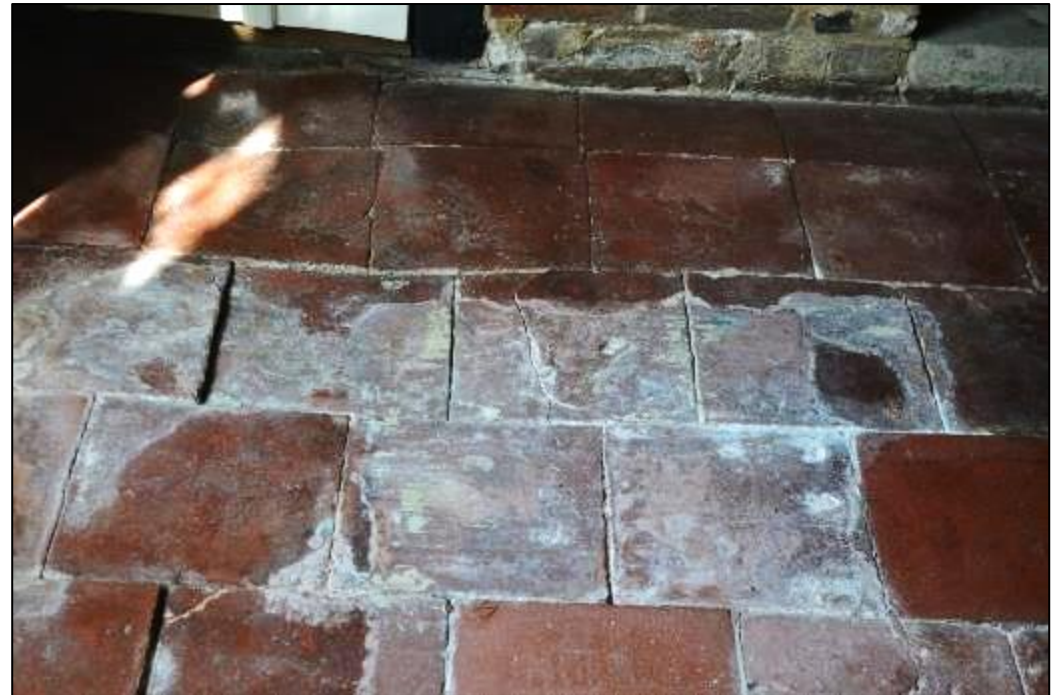
Figure 26: Exposed timber framing and panels are evident throughout the reception room, (right) detail of salt efflorescence – which in itself is a sign of excessive ground water
