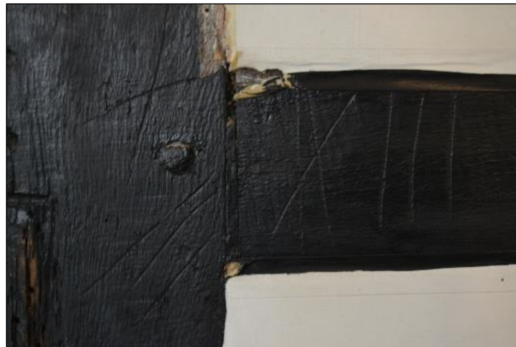
Figure 41: (left) Exposed timber framing and panelling, (right) example of carpenters marks found on timbers throughout the house
