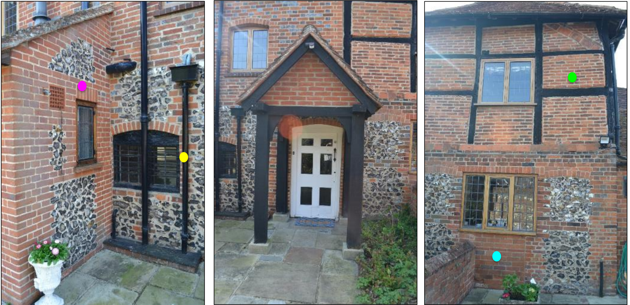
Figure 20: Details of east elevation- (left) 20 th century extension now boiler room (highlighted in pink), surviving single glazed leaded window (highlighted in yellow), (centre) details of 20 th century porch, (right) evidence of potential location of former doorway (highlighted in blue), exposed timber framing thought to be contemporaneous to the adjacent kitchen extension (highlighted in green)
