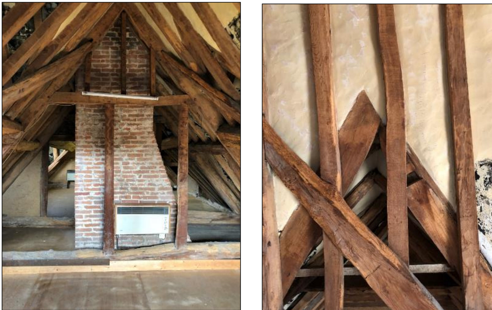
Figure 49: (left) View of internal roof space and central chimney stack, (right) example of modern infill plaster which has been attempted in various locations within the attic
