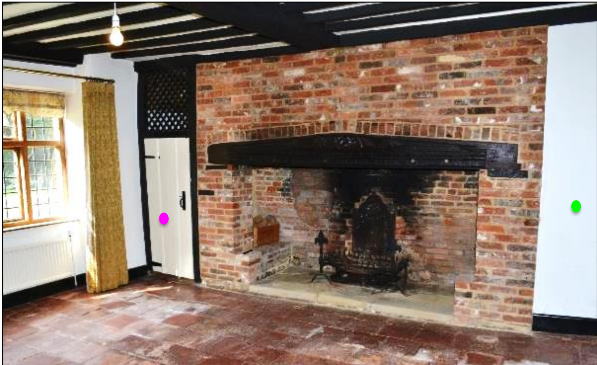
Figure 24: Tudor fireplace in reception hall with moulded timber lintel- note the cupboard to the left (highlighted in pink) and the location of a former door to the right-now blocked (highlighted in green)
