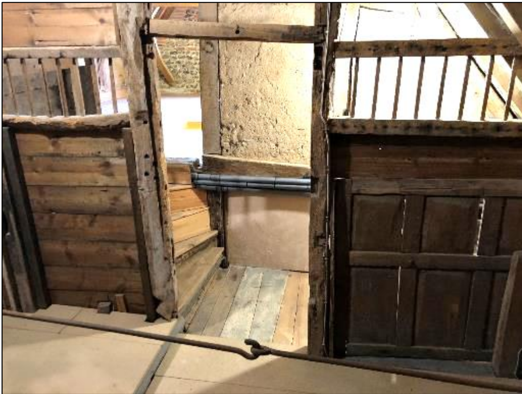
Figure 45: (left) Note the different elements- agricultural and formal- that create the timber partition, (right) view of internal roof structure of central gable along the eastern elevation
