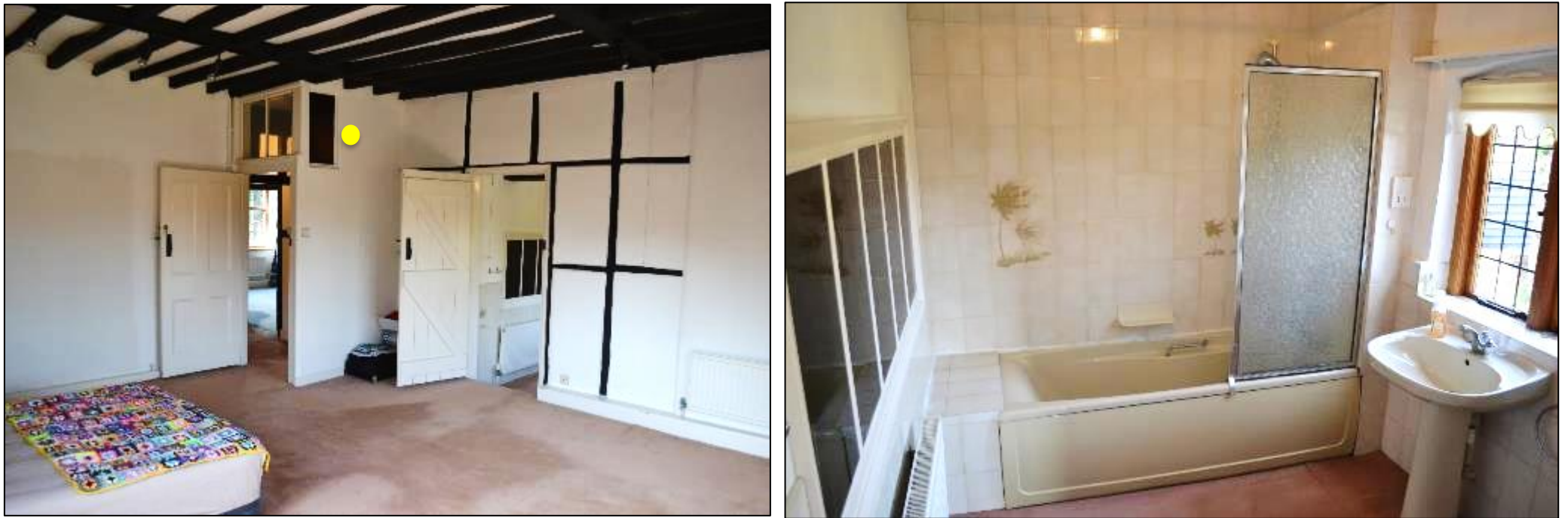
Figure 36: (left) View of timber framing and panelling- note the glazed panels above the entrance door (highlighted in yellow), (right) view into connected en-suite which shares the stained glass window into the hallway
