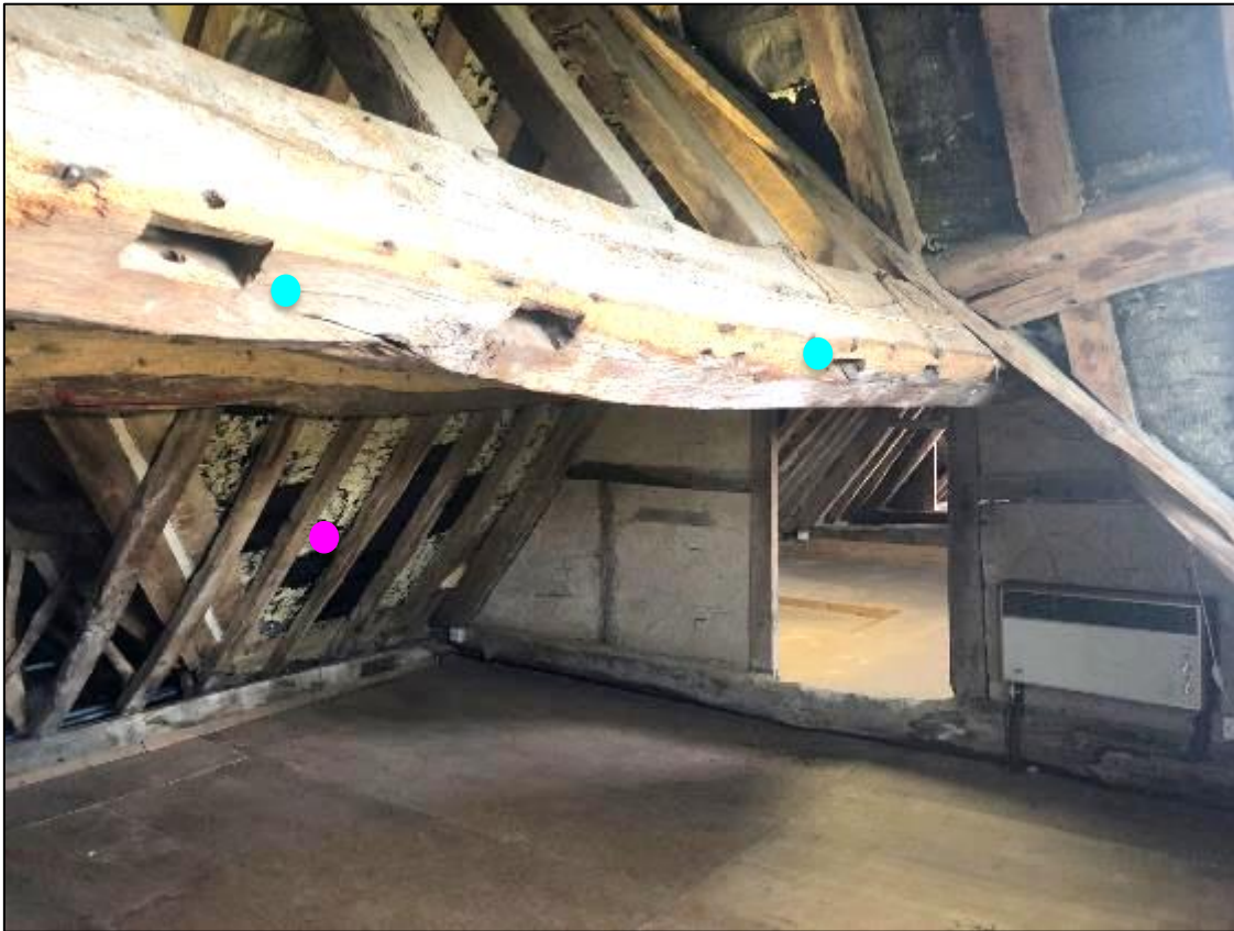
Figure 51: View inside the internal roof void- note the historic plaster panels and 20 th century sarking (highlighted in pink). The details highlighted in blue are evidence to suggest that parts of the timber frame (throughout the entire building-not just the attic) may have been reused from a different building
