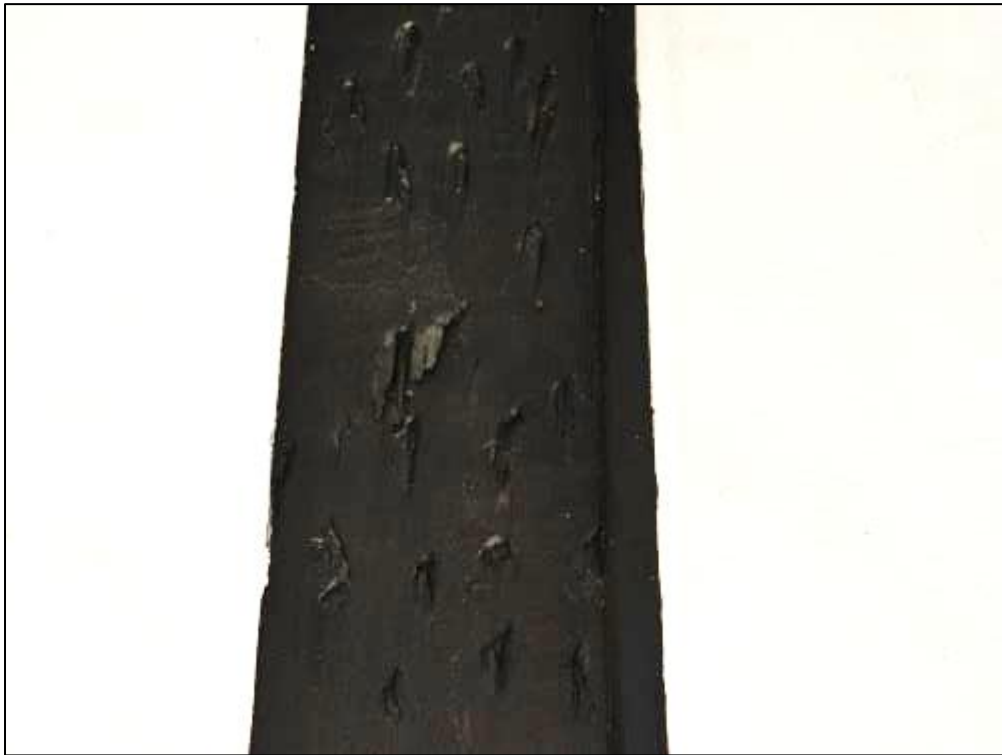
Figure 42: (left) Example of plaster notches found on some of the timber framing throughout the house, (right) brick lined fireplace with timber lintel and adjacent cupboard.
