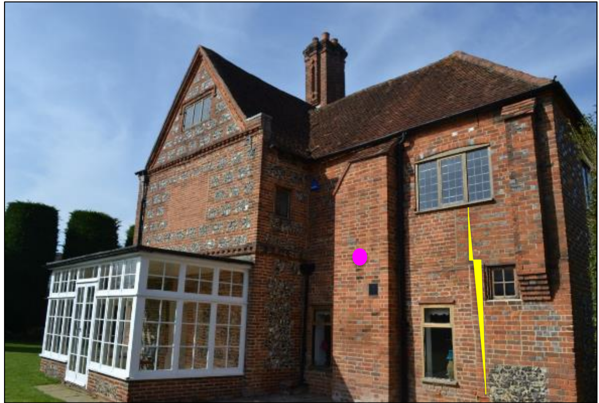
Figure 22: Details of south elevation- (left) note the 1930s garden room/conservatory and blocked off window (highlighted in green), (right) note the remains of a chimney stack that would have been wider than it is at present (highlighted in purple), and 'seam' of where the small 19 th century extension was added (highlighted in yellow)
