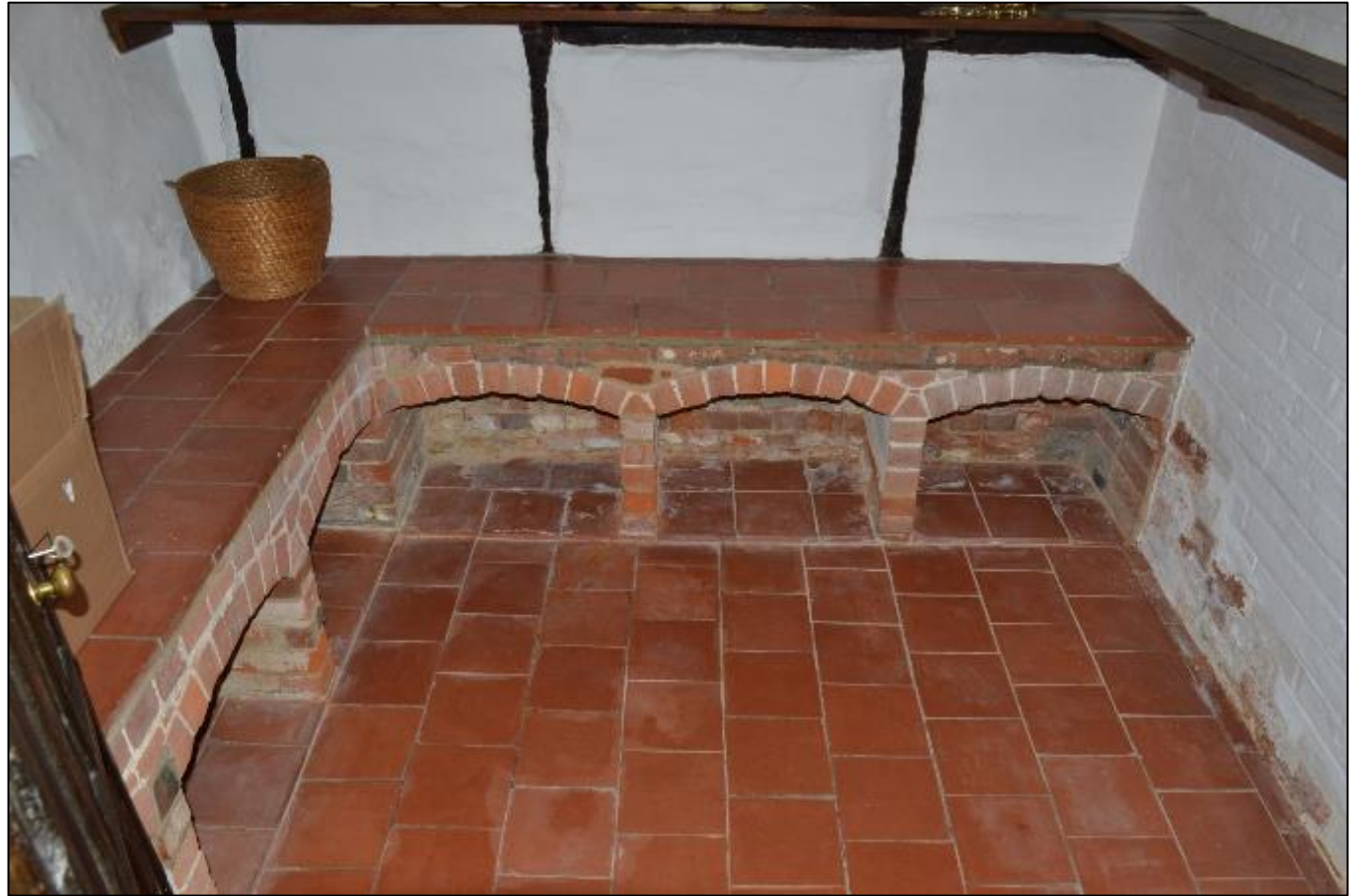
Figure 31: (left) Entrance hall from east doorway, (right) internal view of the wine cellar
