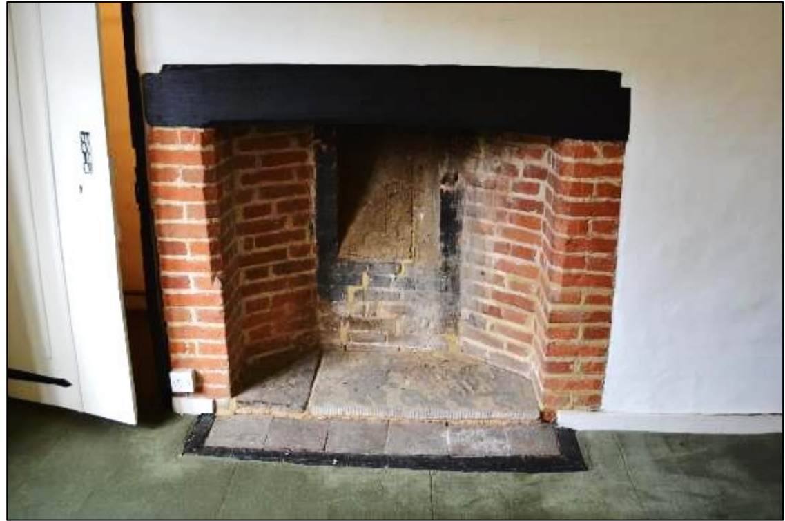
Figure 42: (left) Example of plaster notches found on some of the timber framing throughout the house, (right) brick lined fireplace with timber lintel and adjacent cupboard.
