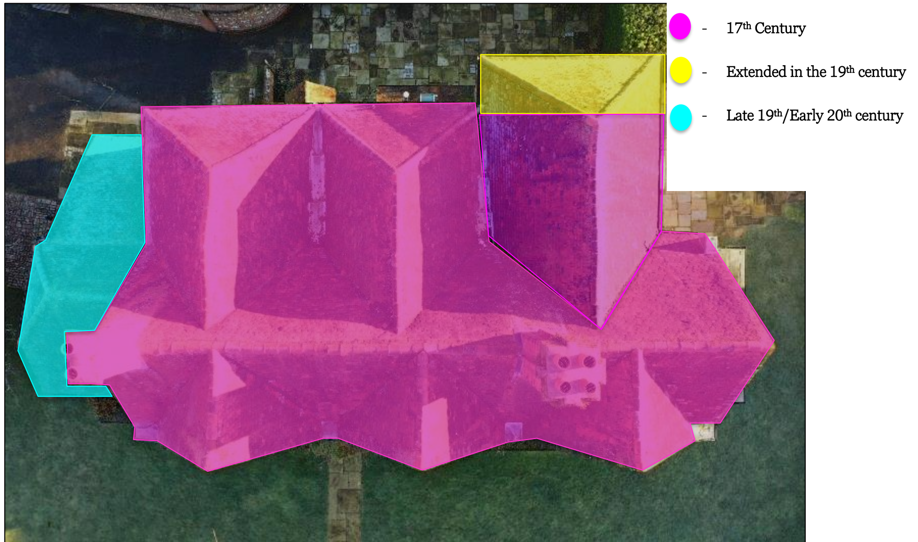
Figure 12: Drone photo of clay tile roof- The entirety of the main roof was re-covered last in a single phase of development, as evidenced by the presence of non-permeable bitumastic sarking felt, which probably took place in the 1970s or 1980s.
