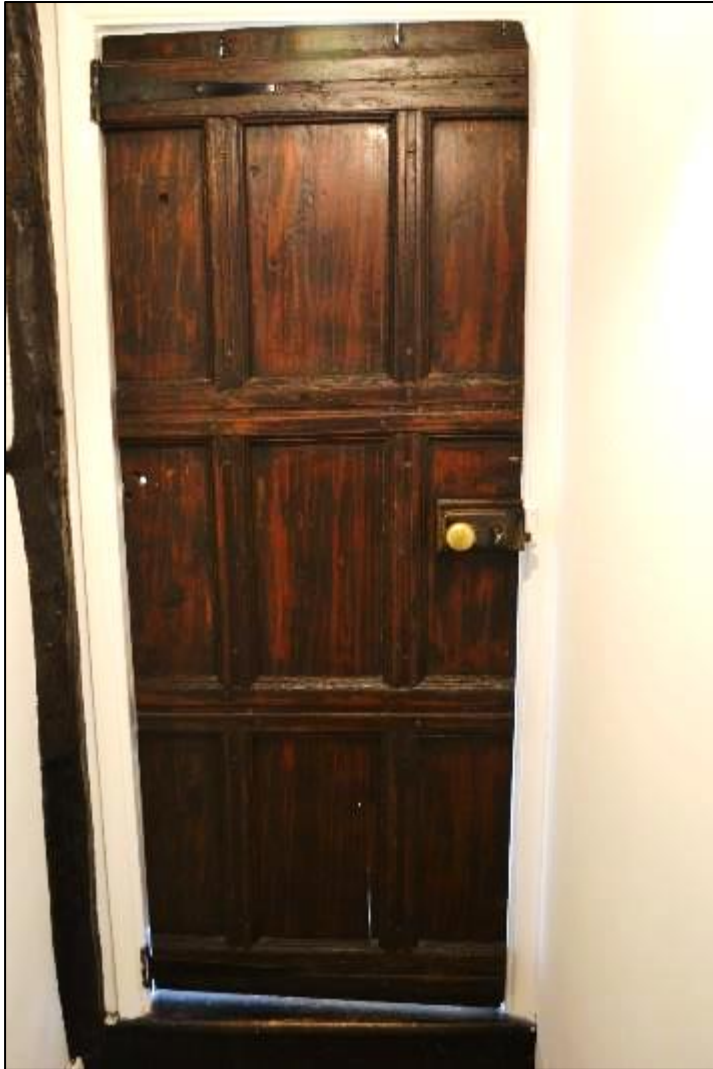
Figure 43: (left) Door separating bedroom 2 from the en-suite- note the door appears to be re-used timber panelling, (right) ensuite bathroom located above 20 th century kitchen extension
