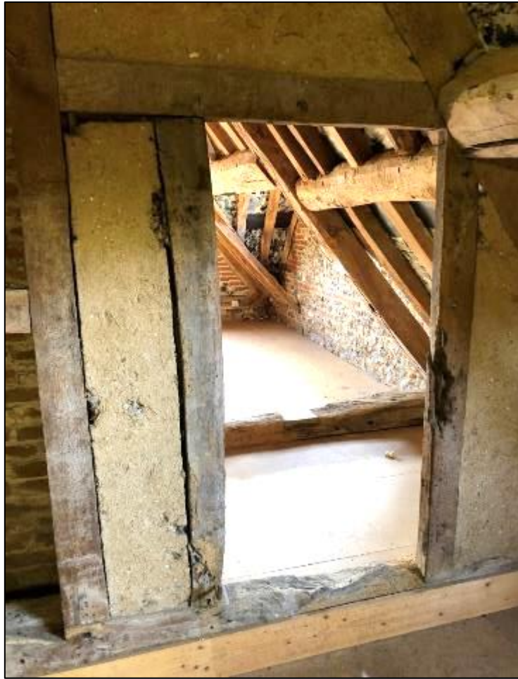
Figure 48: (left) Further examples of historic plaster panels, (right) detail of the lathes thought to be made out of willow upon which the plaster has been applied
