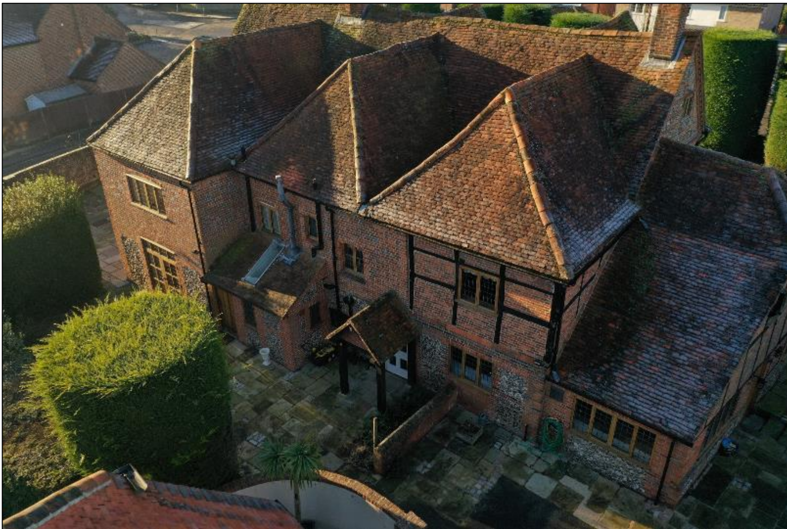
Figure 10: Drone photo overlooking the east elevation
