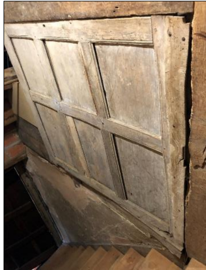
Figure 44: (left) Stairs leading up to attic rooms, (right) example of 17 th century timber panelling (similar to that found downstairs in the principal rooms) being used as a partition
