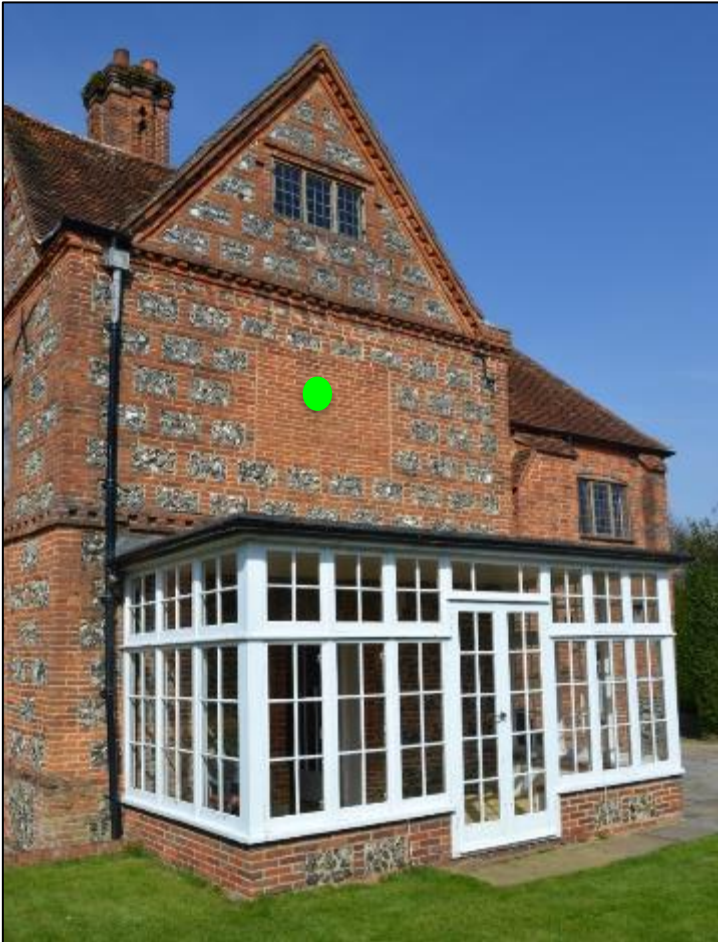
Figure 22: Details of south elevation- (left) note the 1930s garden room/conservatory and blocked off window (highlighted in green), (right) note the remains of a chimney stack that would have been wider than it is at present (highlighted in purple), and 'seam' of where the small 19 th century extension was added (highlighted in yellow)
