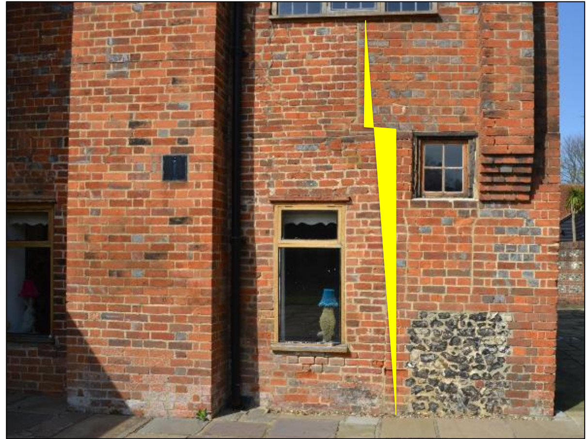
Figure 23: Details of south elevation- it is not entirely clear why the building was extended by such a small amount in the 19 th century (highlighted in yellow)- however it is likely that the chimney stack would have served a further 'service room' before being part removed.
