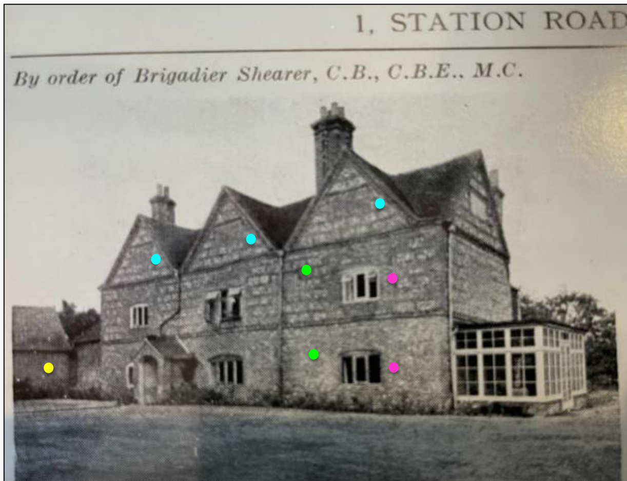
Figure 16: Early 20th Century photograph from Country Life- blocked off windows in the 3 projecting gables now open (highlighted in blue), example of smaller windows in situ at the beginning of the 20 th century- these have been replaced with larger, wider units (highlighted in pink), blocked off window on the first floor under a hood moulding but no evidence of a hood moulding on the ground floor- both now open windows (highlighted in green), evidence of former outbuilding (now demolished) which once ran east-west to the north of the principal building and kitchen (highlighted in yellow)
