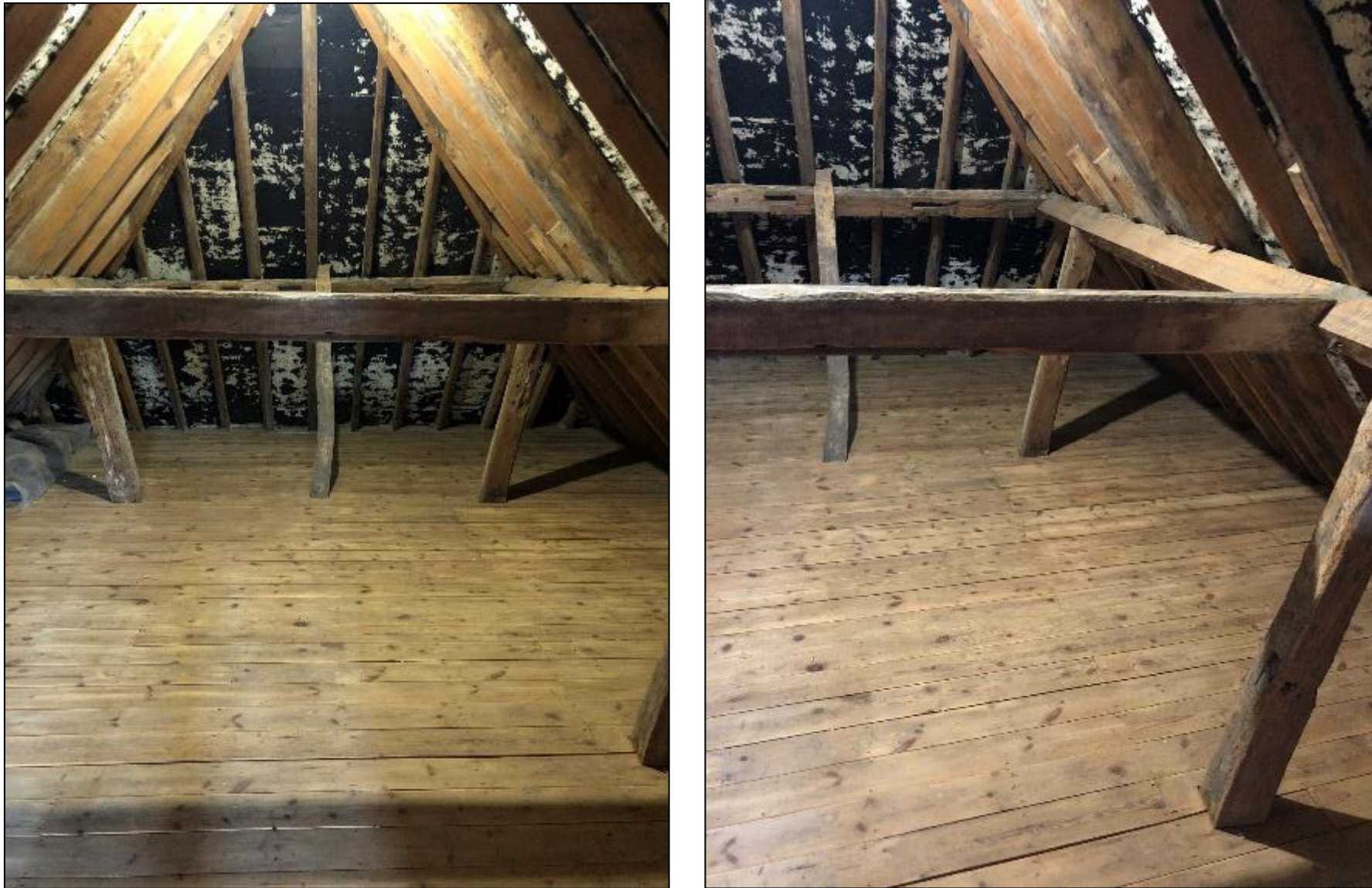
Figure 50: View inside the southernmost gable along the east elevation- note that this has been extended in the 19 th century
