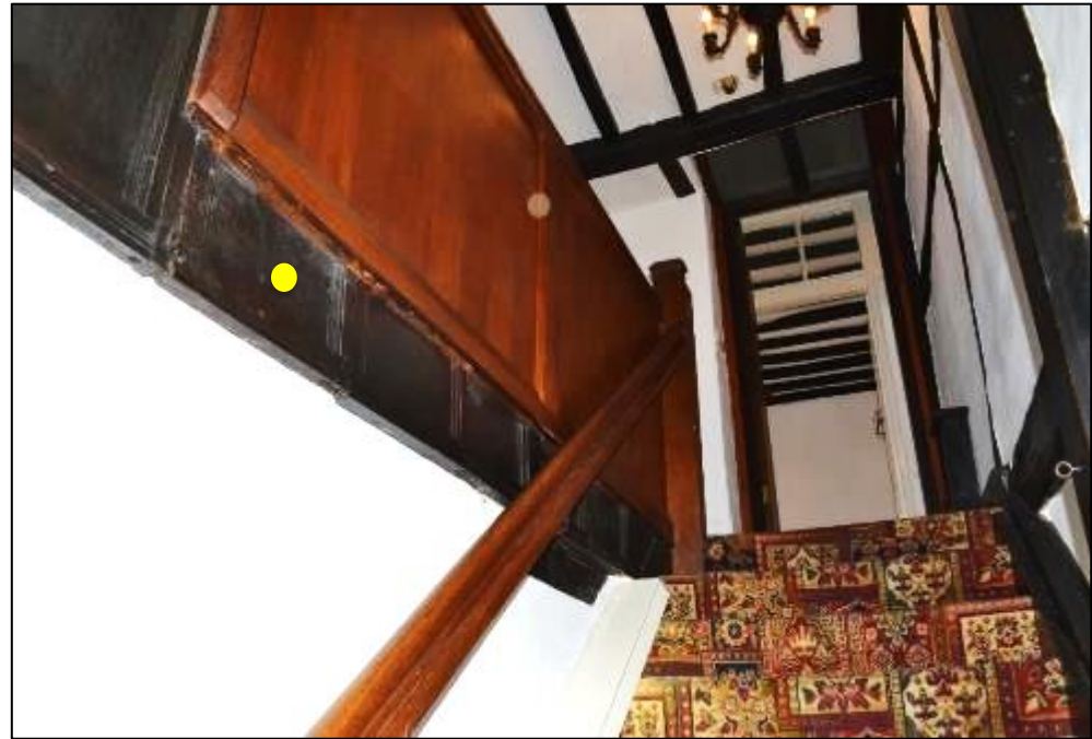
Figure 34: (left) View of hallway leading to the main central staircase which is thought to have potentially replaced an earlier one thought to have been located in the family room, (right) detail of timber wall panelling reused along the staircase as some of the panels are now drawers (highlighted in yellow)
