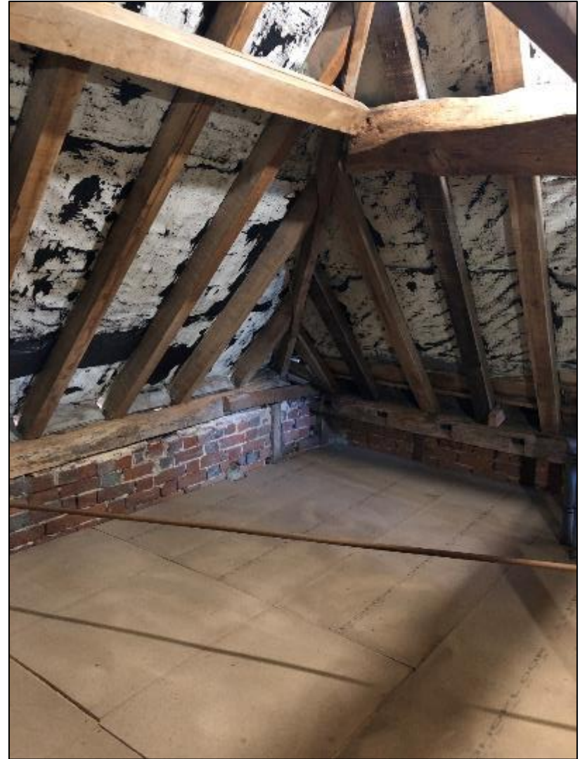
Figure 45: (left) Note the different elements- agricultural and formal- that create the timber partition, (right) view of internal roof structure of central gable along the eastern elevation
