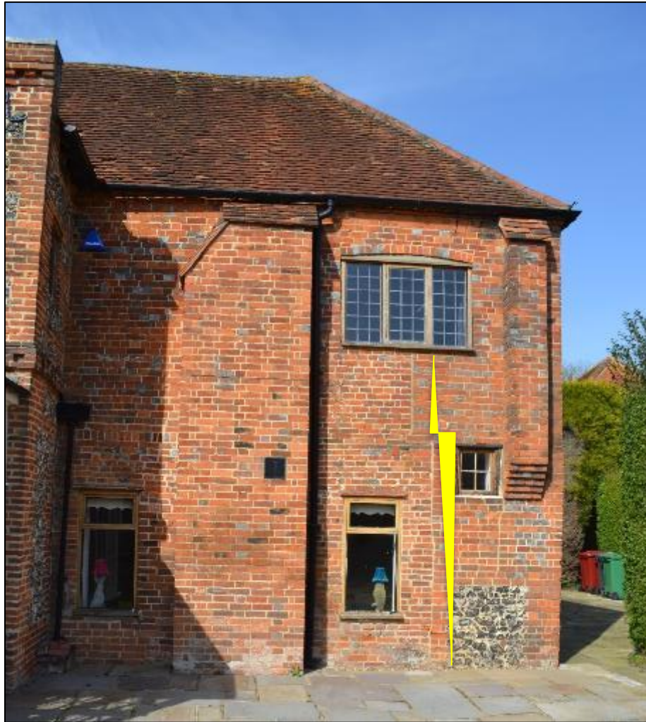
Figure 23: Details of south elevation- it is not entirely clear why the building was extended by such a small amount in the 19 th century (highlighted in yellow)- however it is likely that the chimney stack would have served a further 'service room' before being part removed.
