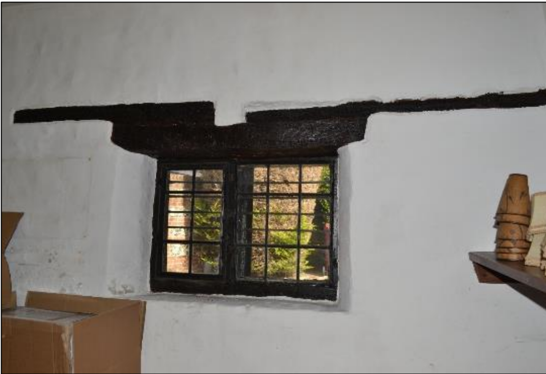
Figure 32: (left) Original timber single glazed leaded window, (right) example of one of the many timber panelled doors within Old Grove House
