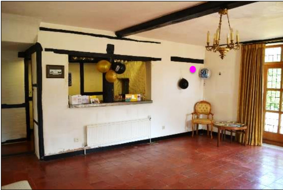
Figure 30: Bar located within the family room, blocked off doorway (highlighted in pink) which would have led out to what is now the location of the boiler room
