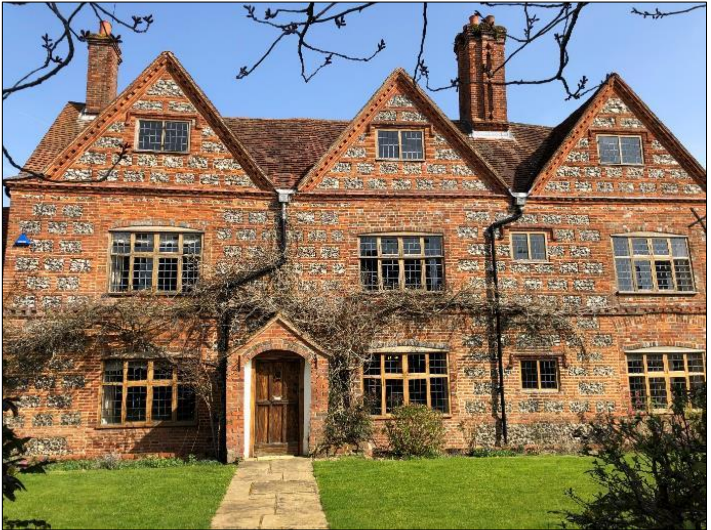
Figure 15: West elevation of Old Grove House
