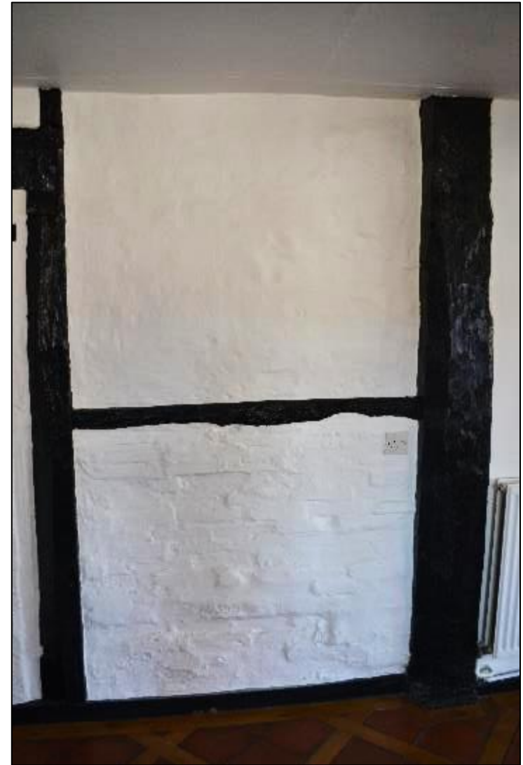
Figure 33: (left) View of kitchen from north-western corner of the room, (right) timber panelling and brick infill along wall shared with the reception room
