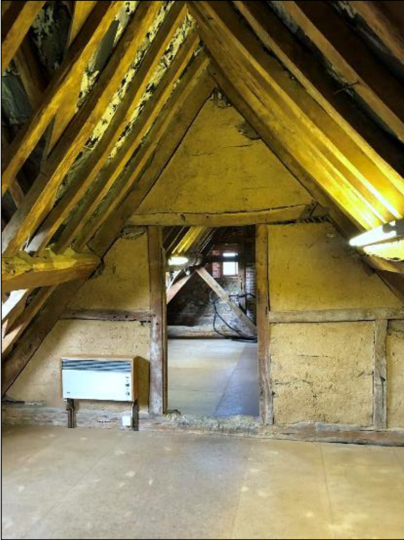
Figure 46: (left) Internal view of central roof space- note the original plaster infill panels, (right) example of where the roof structure has been repaired and new timbers spliced in
