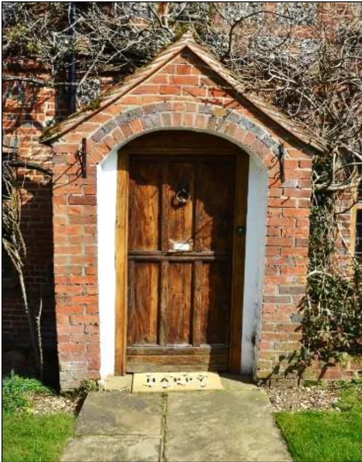
Figure 17: Details of the west elevation- (left) 20 th century porch inset with 17 th century door, (right) when compared to Figure 16 the fenestration alterations become clear, the inserted two light casement windows under hood mouldings (highlighted in green), and the 4 light mullion and transom windows which have been increased in size from the early 20 th century
