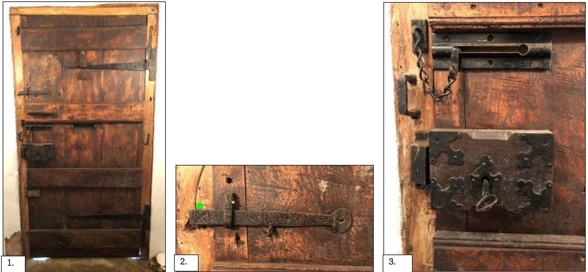
Figure 25: Detail of porch door- 1. 17 th century plank timber door, 2. Detail of iron latch on door-interestingly this design with a 'X' is seen throughout the house on other latches, 3. Detail of further ironwork on the door
