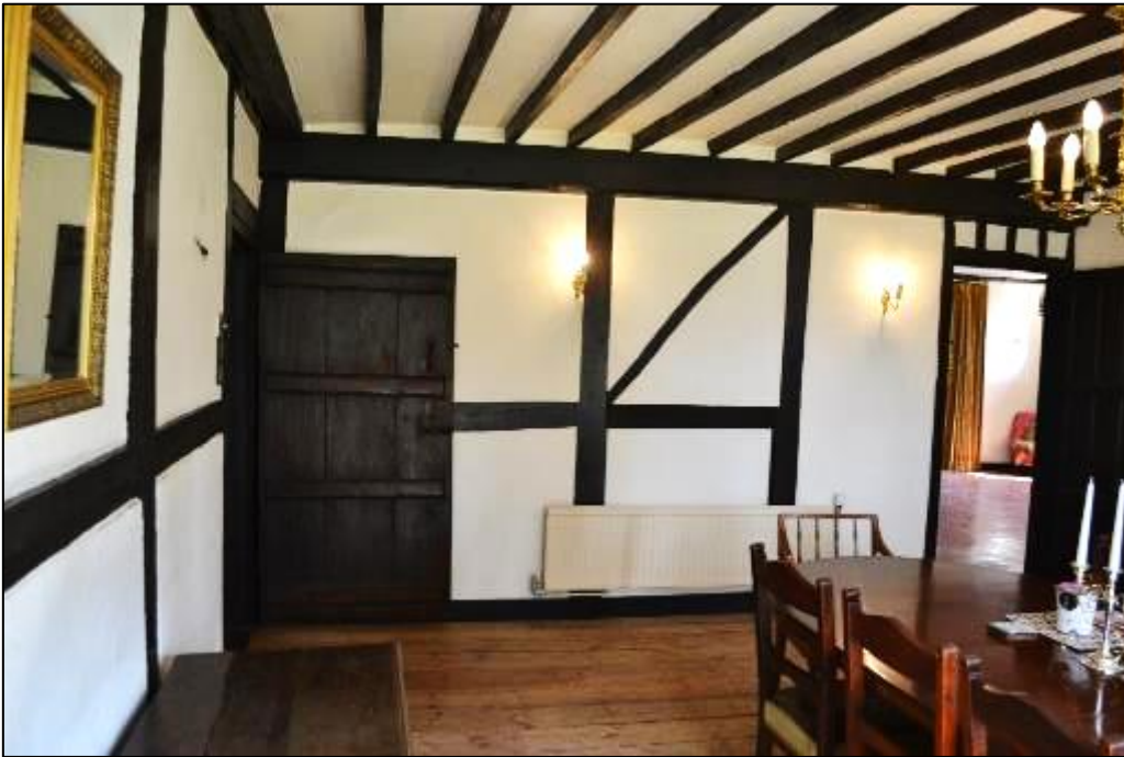
Figure 27: Exposed timber framing throughout, (right) remains of 17 th century timber panelling (highlighted in pink) and large Tudor depressed brick arch fireplace and moulded mantel with masked brackets (highlighted in yellow)
