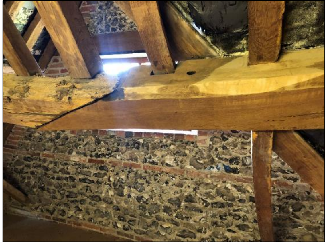
Figure 46: (left) Internal view of central roof space- note the original plaster infill panels, (right) example of where the roof structure has been repaired and new timbers spliced in
