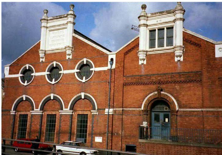
Tram depot power house
