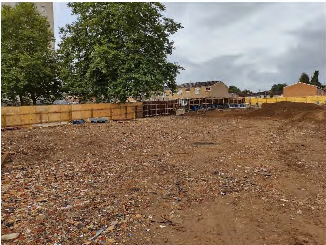
Plate 4 – View southwest across the site
