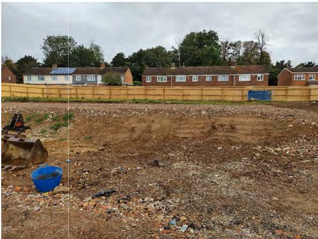
Plate 2 – View north across the site
