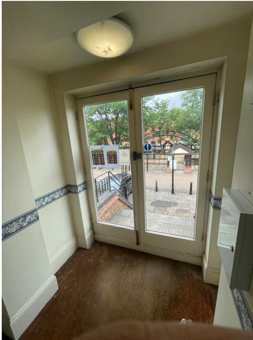
Photograph 3: Rear access door and hallway area. Existing door unit and furniture to be retained. Light fitting to be cleaned and retained. Key cupboard to be replaced with aged brass equivalent to maintain consistent internal finishes.
