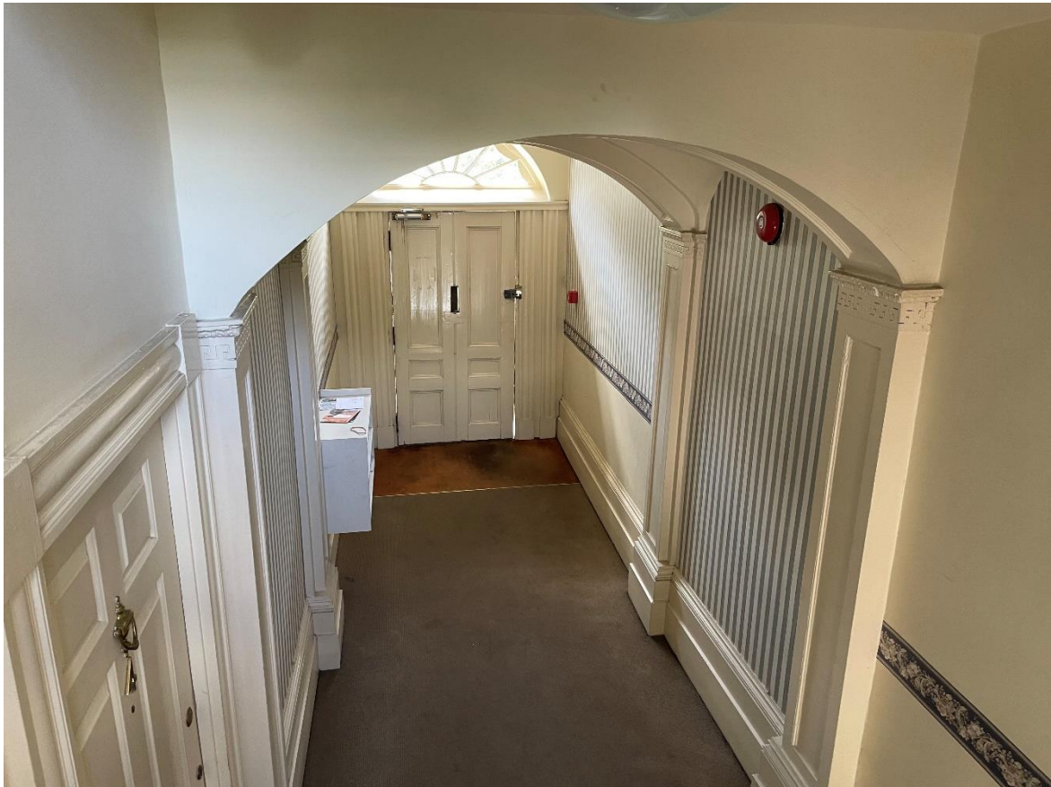
Photograph 2: Main entrance hallway. Note there are to be no alterations to the existing wall or ceiling relief, and no changes to timber joinery detailing such as skirting and architraves.
