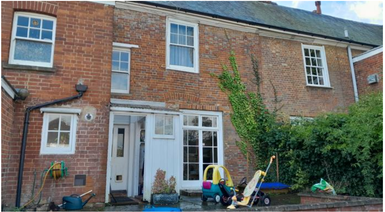
Fig 1. Rear of 156 Castle Hill. Site photo taken by Case Officer on 26/10/2022
