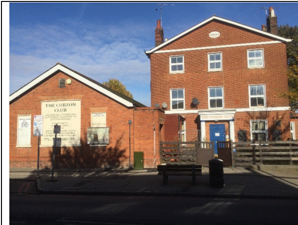
Photograph 1. The south facing elevation of the 362 Oxford Road.
