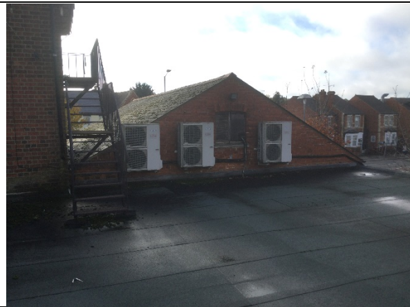
Photograph 8. The flat roof section upon the single story area to the north of the building.
