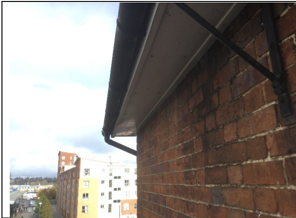
Photograph 7. The well fitting PVC soffits fringing much of the roof.
