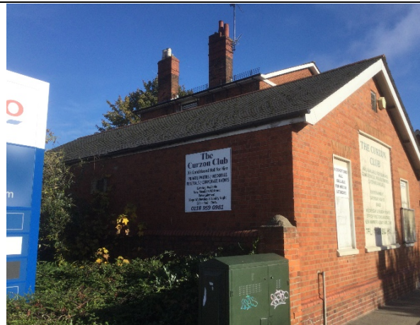
Photograph 2. The southwest facing elevation of one of the single story sections of the building.
