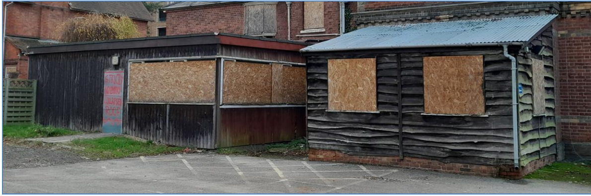
Fig 3. Rear of 3 Craven Road, existing rear extension (left) to be replaced and lean-to (right) to be removed pictured. Photo taken by Case Officer on 11/11/2022.
