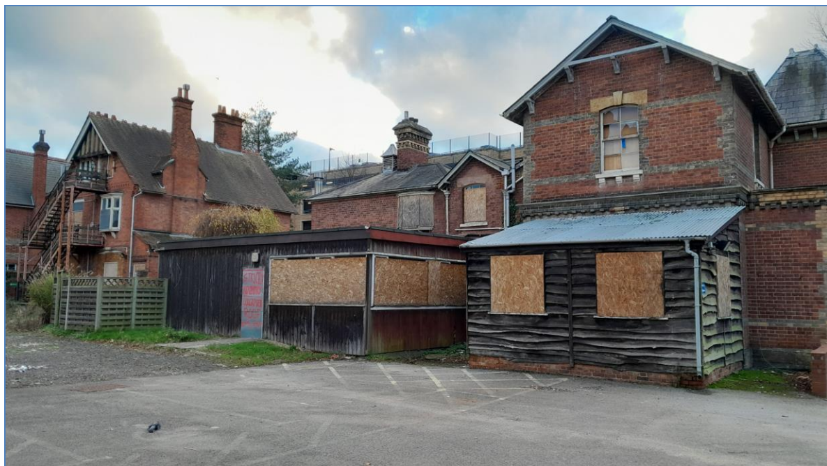
Fig 2. Rear of 3 and 5 Craven Road. Photo taken by Case Officer on 11/11/2022.
