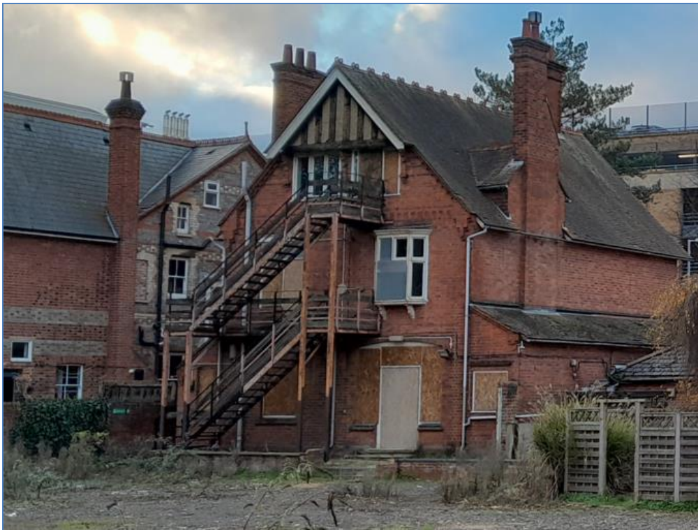
Fig 4. Rear of 5 Craven Road, external staircase to be removed pictured. Photo taken by Case Officer on 11/11/2022.
