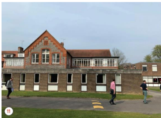
Photograph of the existing building
