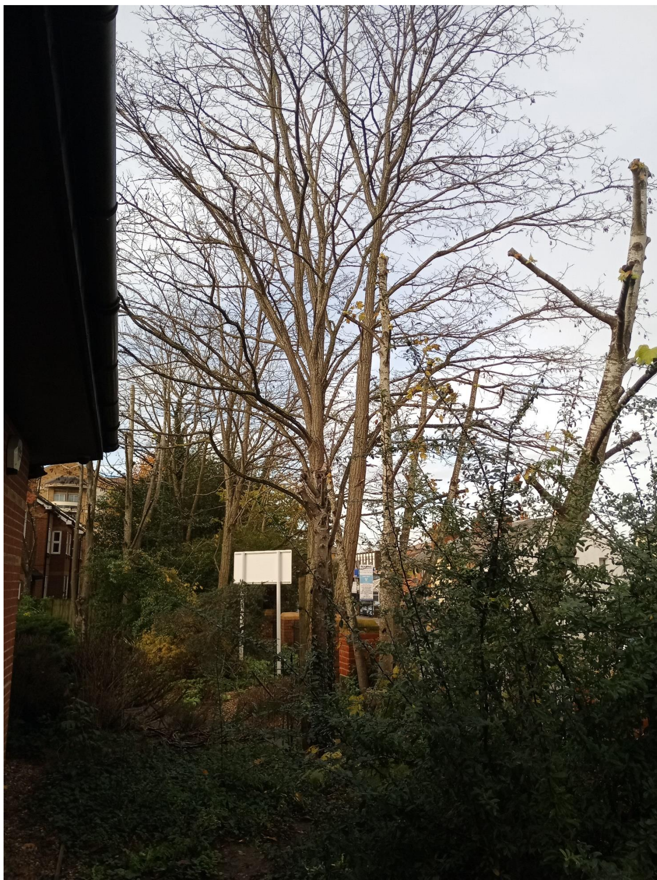
Looking along the side of the building towards the bus stop
