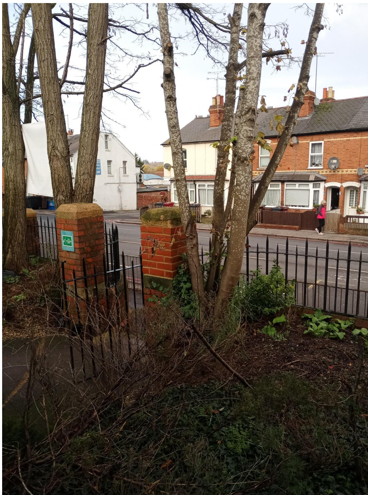
Tree No. 5 – Note repaired brick work adjacent
