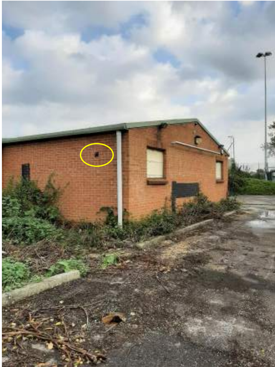
Plate 2.1: Site 1 at the eastern end of the former driving range building
