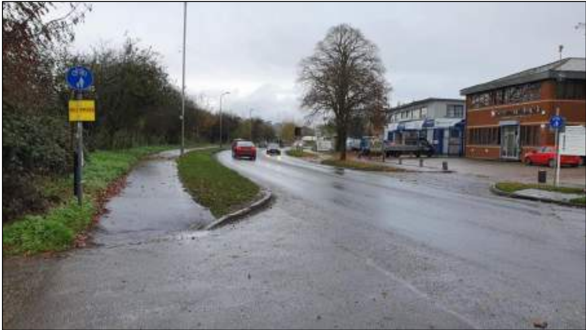
Figure 2.5 – Richfield Avenue east in vicinity of site access
