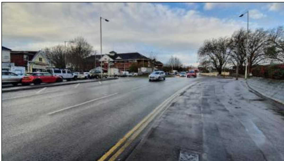
Figure 2.7 – Caversham Road north toward River Thames
