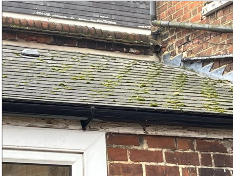
Photograph F Close-up of the rear slate roof of the extension
