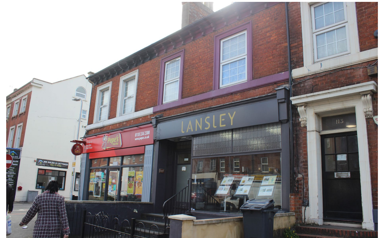
Largely intact historic shopfront at no. 111, with Early-Victorian sash windows
