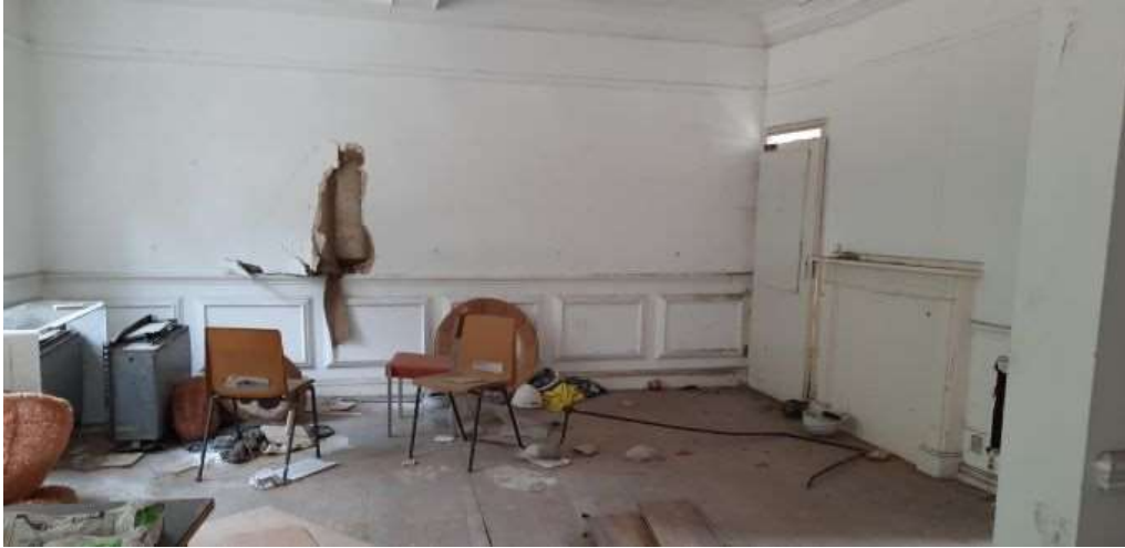
Picture 2: Former interior door on first floor now open to exterior with gap above. Superficial damage to wall providing no potential roost space.
