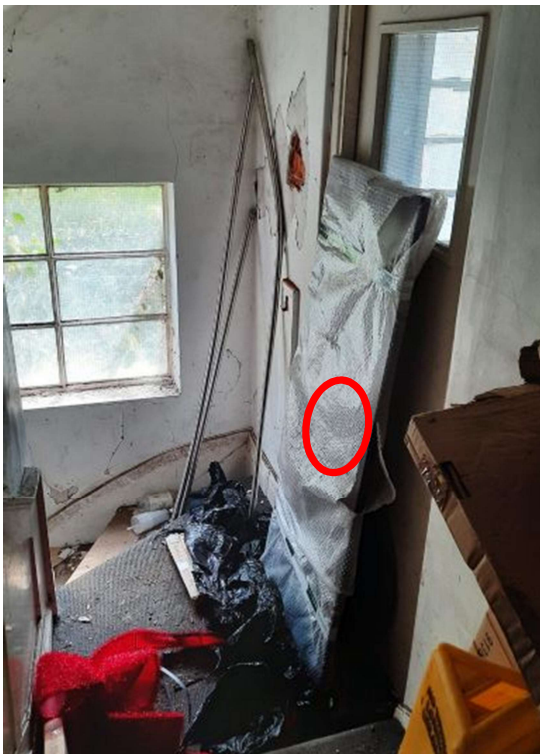
Picture 1: Bubble-wrapped board leaning against interior door on ground floor where a single bat dropping was identified, attached to the rear (approximate location indicated by the red circle).
