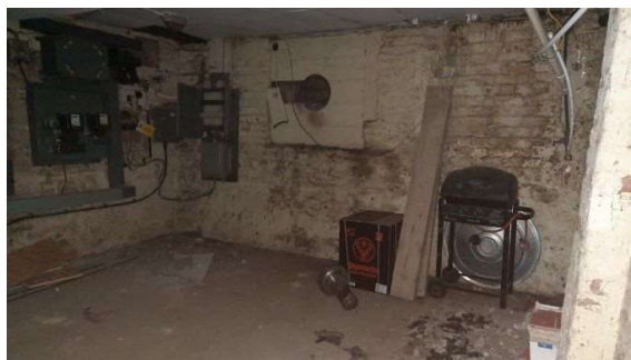
Picture 9 and 10: Basement
