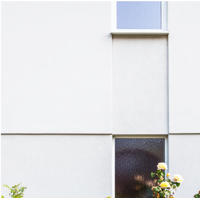
REFERENCE DESIGN: Rainscreen cladding with high-quality render finish
