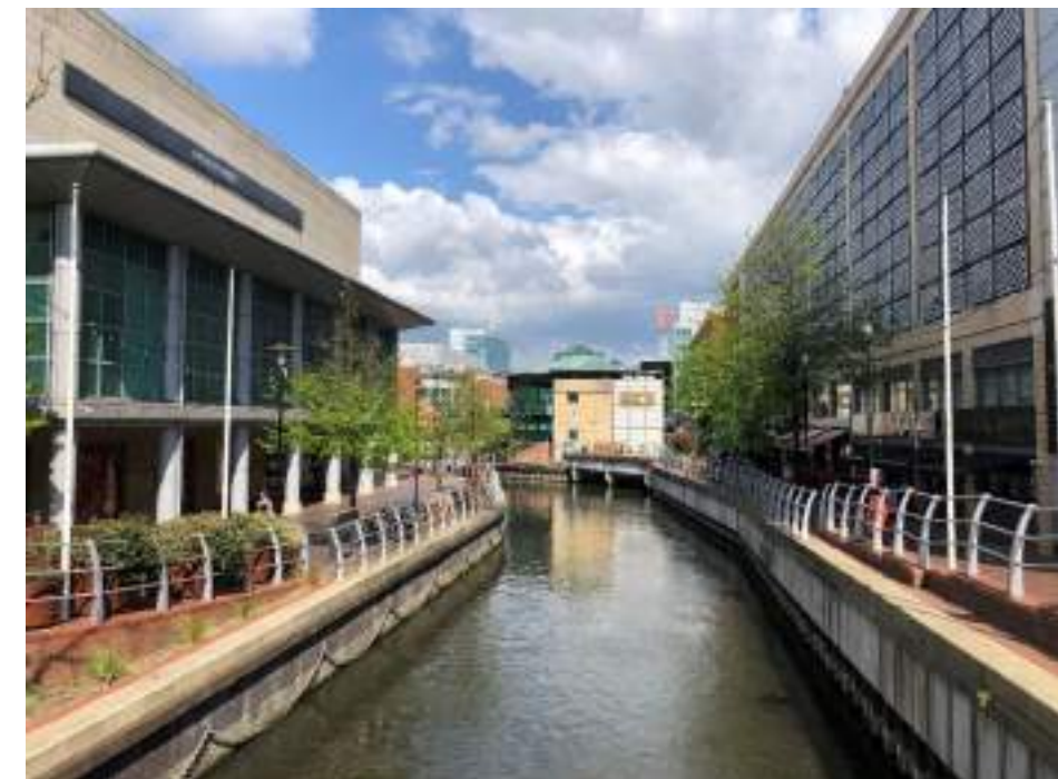
Figure 3.8: Photograph of Site as seen from the west and Bridge Street bridge along River Kennet (2022)
