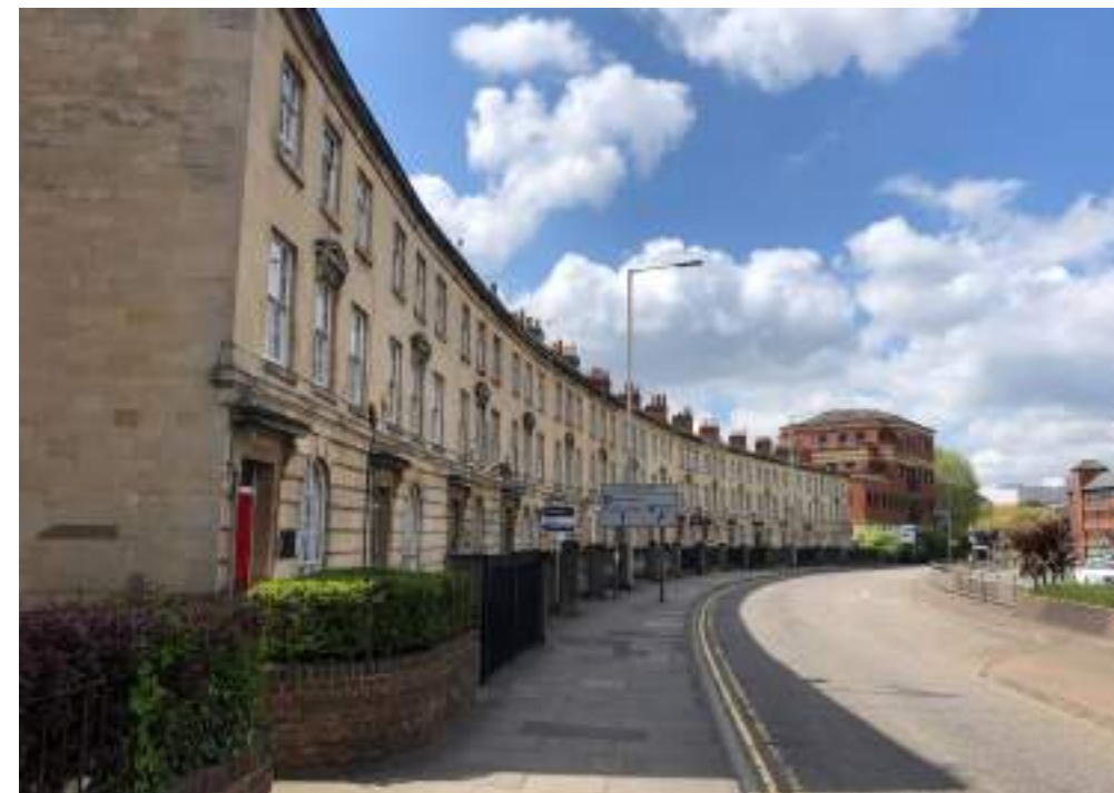
Figure 3.17: View of Nos. 24-52 Queen's Crescent
