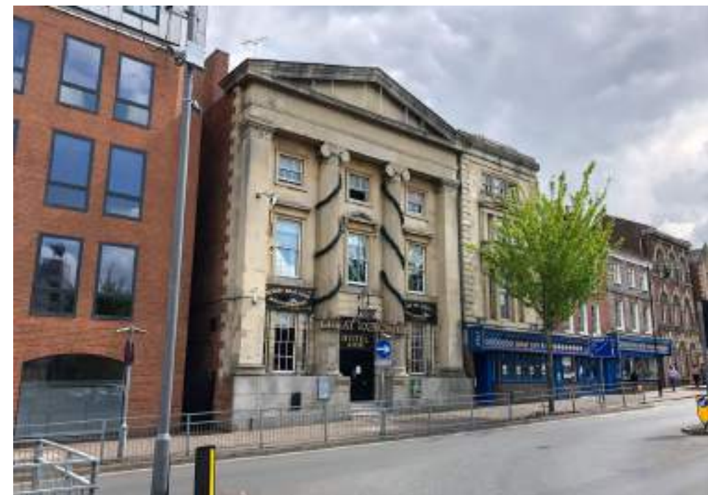
Figure 3.13: View of Nos. 33-41 London Street
