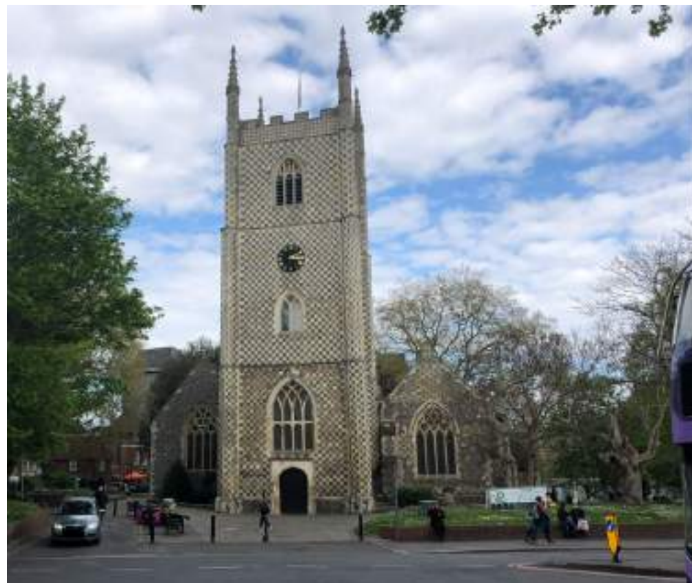
Figure 3.22: View of Church of St Mary, St Mary's Butts
