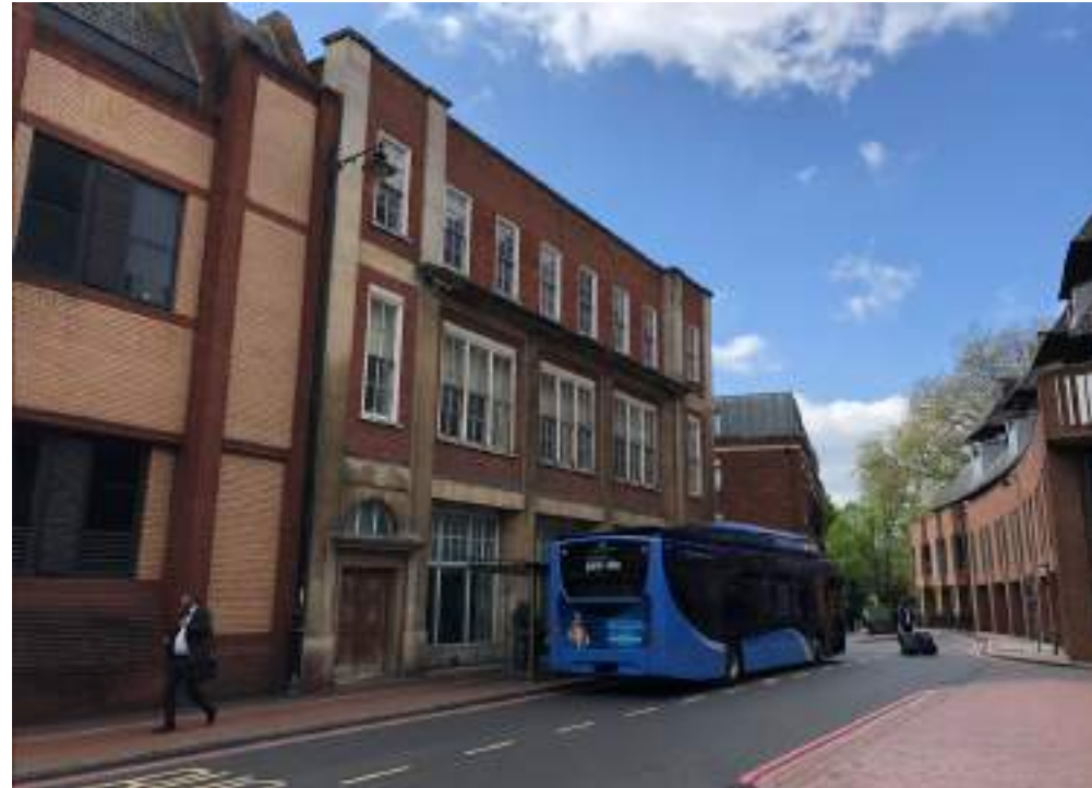
Figure 3.21: View of Telephone Exchange, Minster Street
