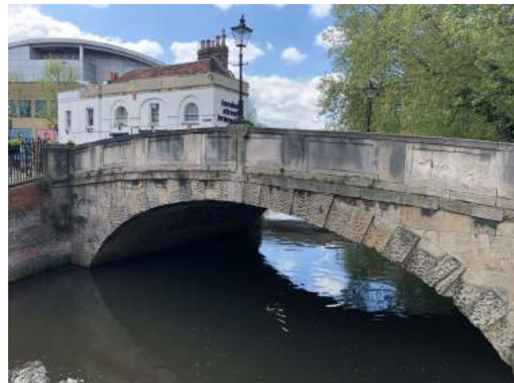
Figure 3.12: View of High Bridge from the waterside
