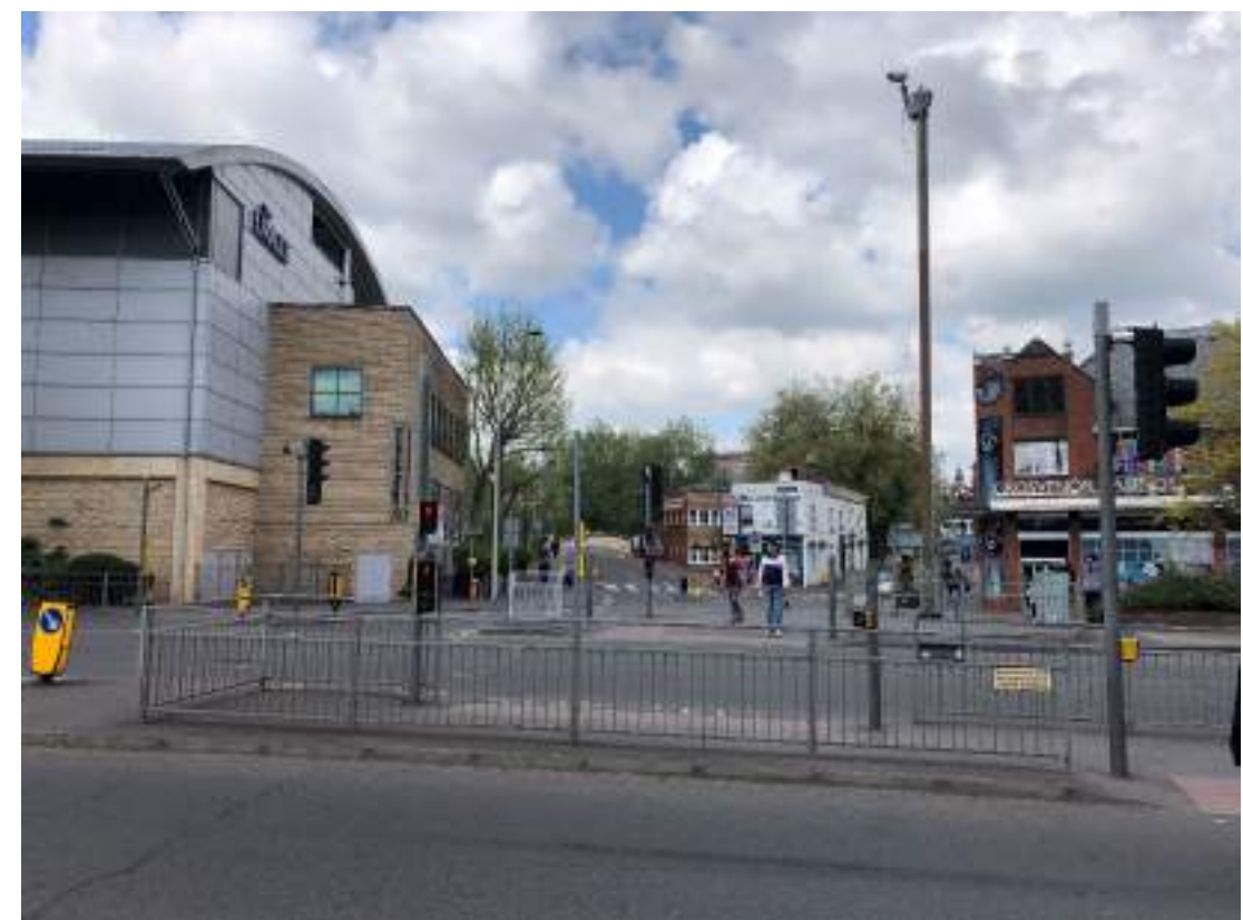
Figure 4.8: View looking north at the pedestrian crossing of the IDR and gateway / conjunction of High Bridge Yield Hall Place bridge
