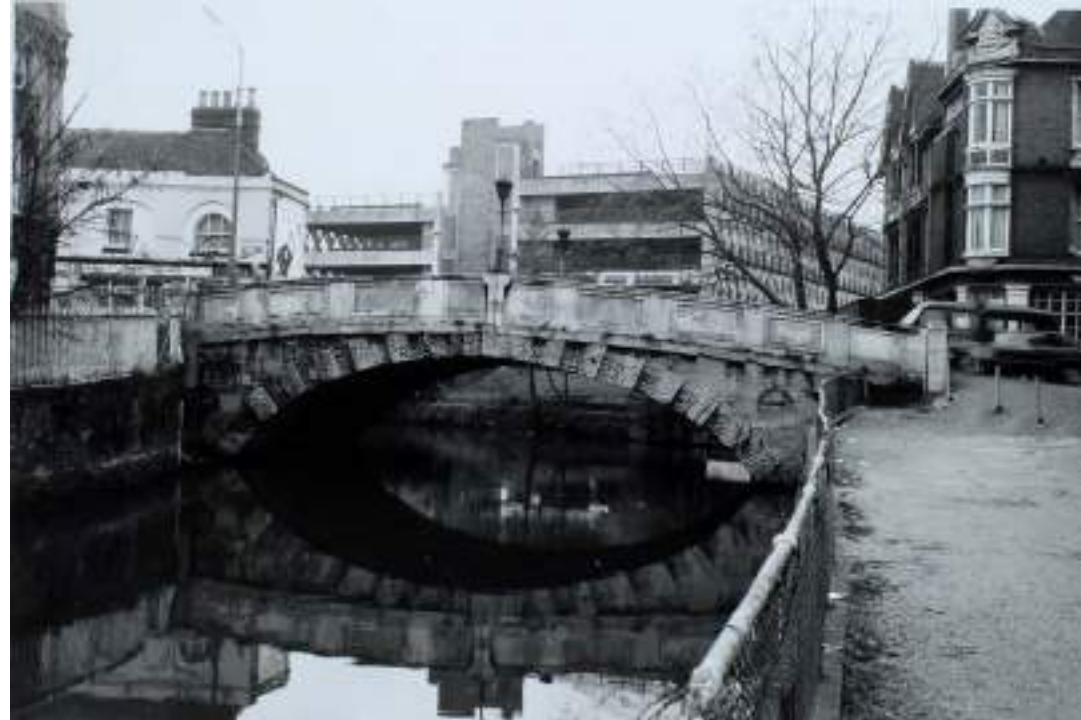
Figure 3.4: Photograph of the High Bridge from the east looking west towards the Site, dated 1981 (prior to The Oracle redevelopment) 4
