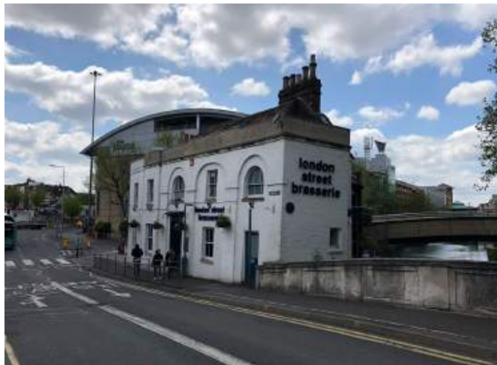
Figure 3.10: View of Nos. 2-4 London Street
