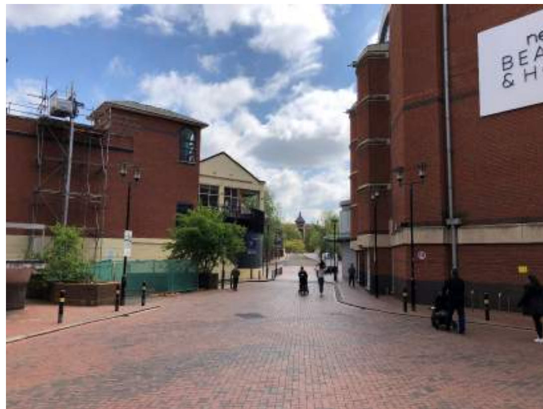
Figure 4.7: View looking south along Yield Hall Place and bridge to the east side of the Site
