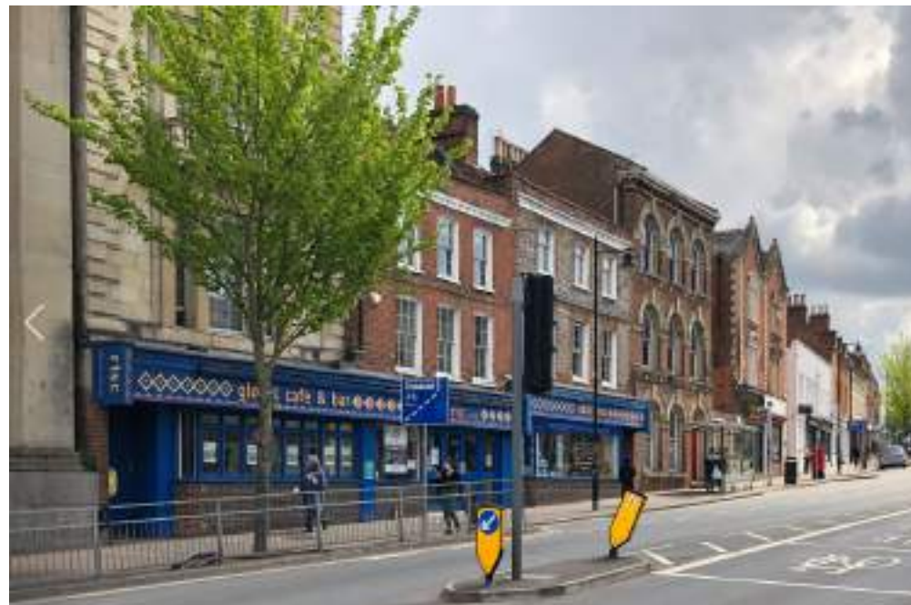
Figure 3.14: View of Nos. 35-41 London Street
