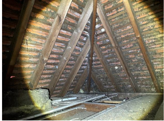
Photo 6 – Building 2, inside void
