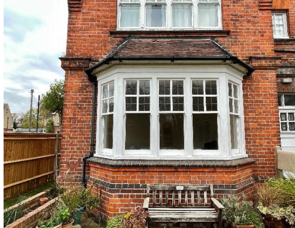
Photo 1 – Building 1, bay window
