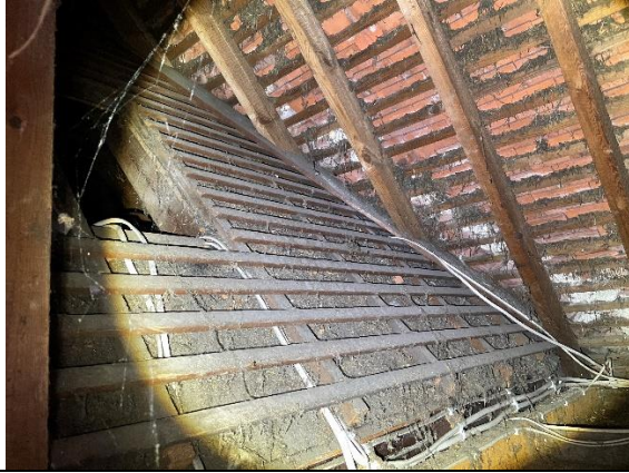
Photo 5 – Building 2, inside void
