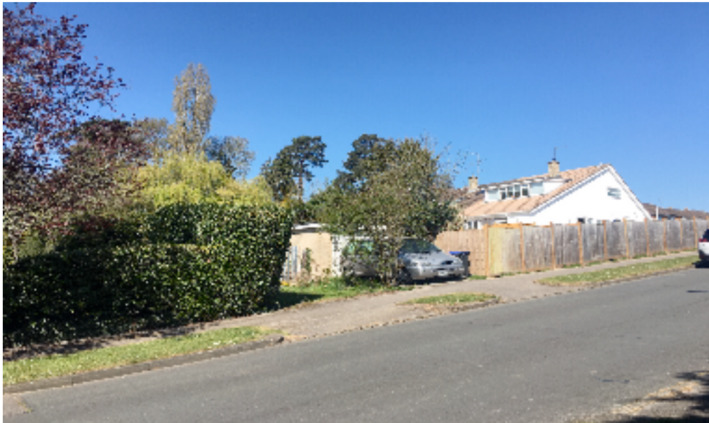
Fig v. East boundary view of the site showing the existing garage and recessed sub station site.
