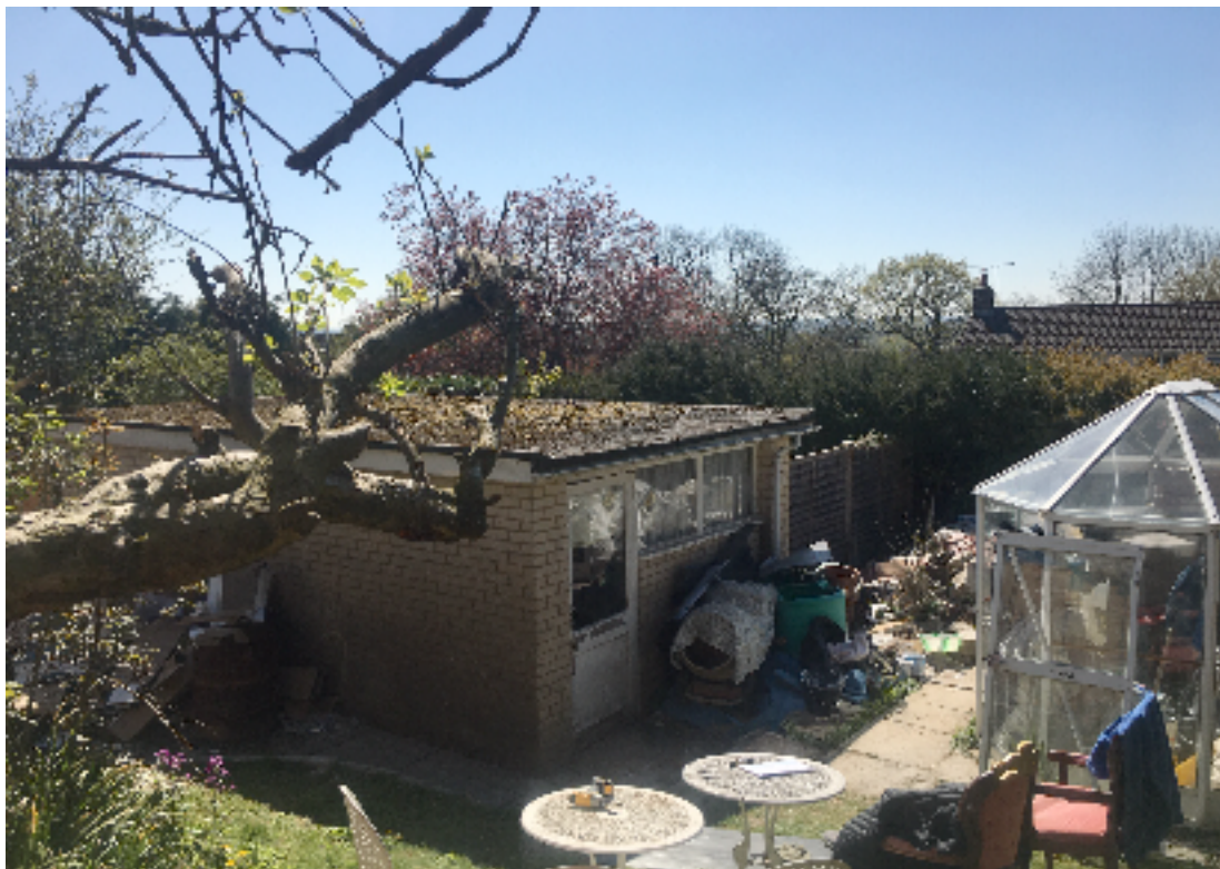
Fig ii. View from within the site of the single storey existing garage and outbuilding
