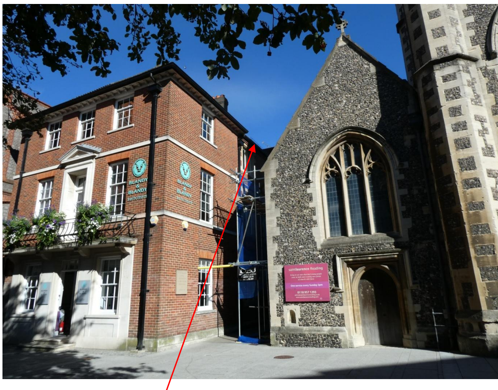
Fig 2: West end of St Laurence's Church and adjacent property to the north where tile guards have also been fitted
