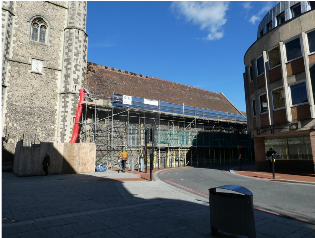
Fig 1: South side of St Laurence's Church illustrating proximity of the church to the footpath and road
