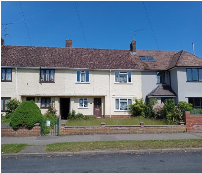
Figure 1: Existing front elevation (site visit - 27 th May 2022).
