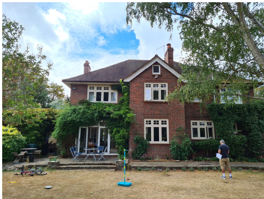
Existing rear elevation (extension to replace garage to left overgrown with planting)
