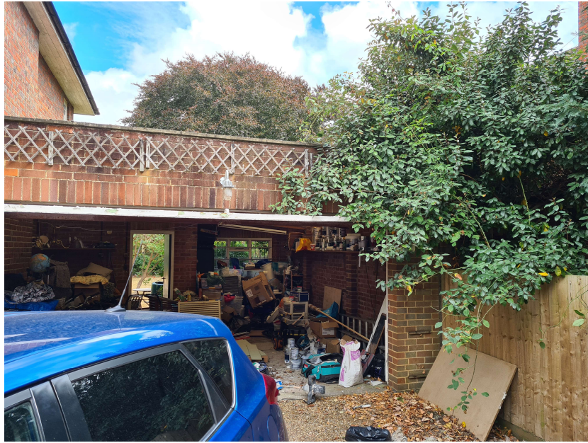
Garage to be replaced
