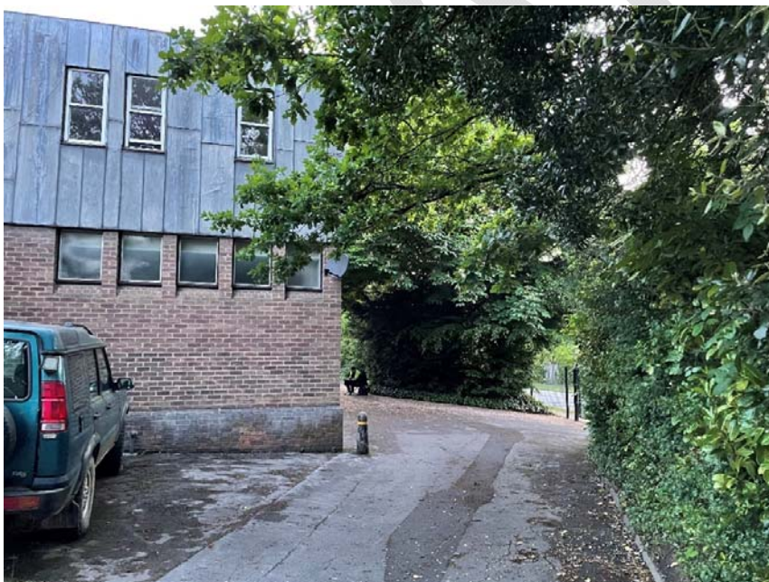
Plate 2 Surveyor position to north of 2-storey structure
