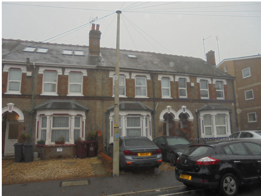
Photo 1 – View of the front of the property
