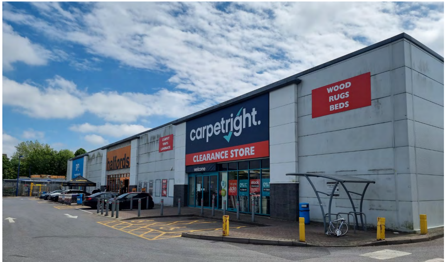
Figure 2: Existing Retail Terrace from the Car Park
