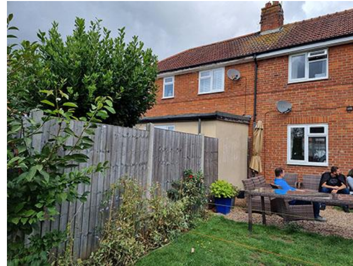
Existing rear extension at No. 26
