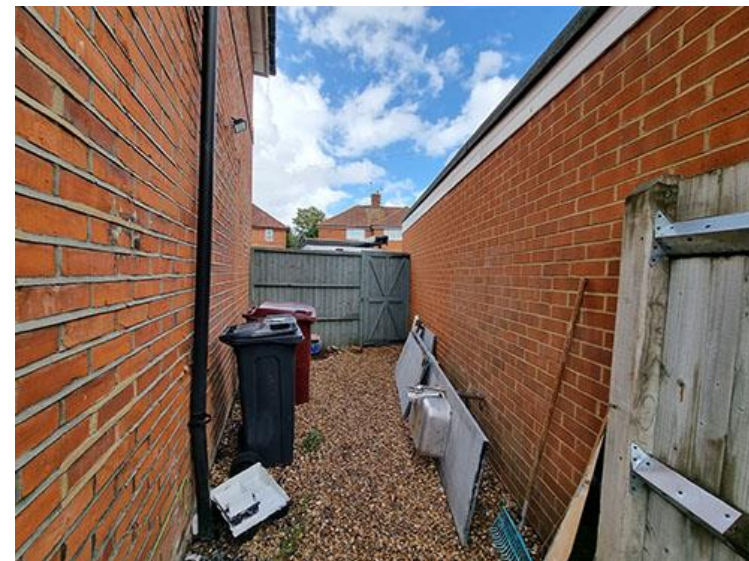
Existing view to front gate
