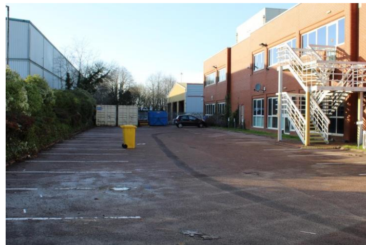
Looking west along southern boundary.
