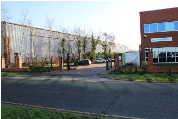
Existing site entrance served from Bennet Road.
