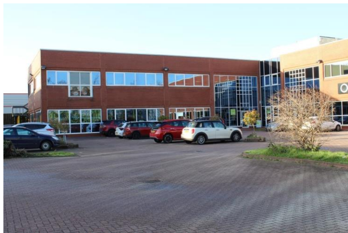
Rear of Block 1 facing inner courtyard.
