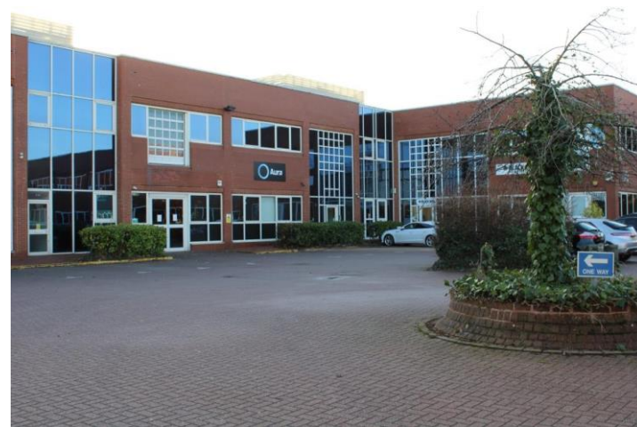
Front of Block 2 facing inner courtyard.
