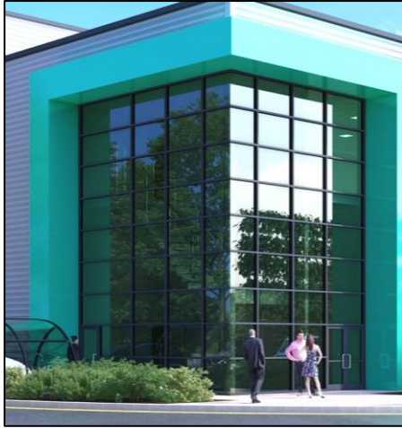
Curtain walling (External)
