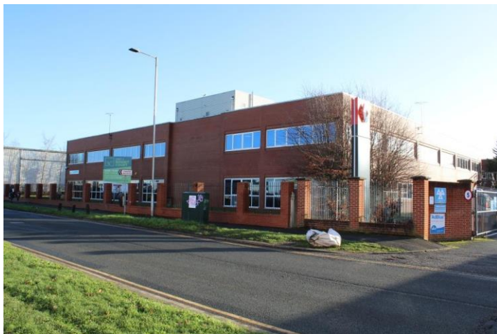
Site frontage from Bennet Road.
