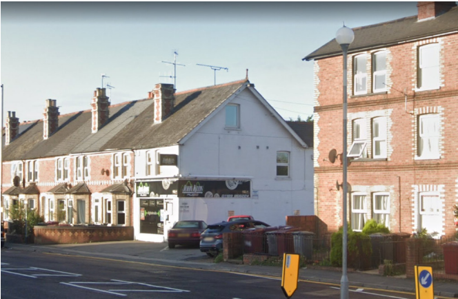
View facing south from Basingstoke Road showing parts of the site and entrance to the rear of the site. The proposal would be almost entirely concealed from this perspective on the public highway.
