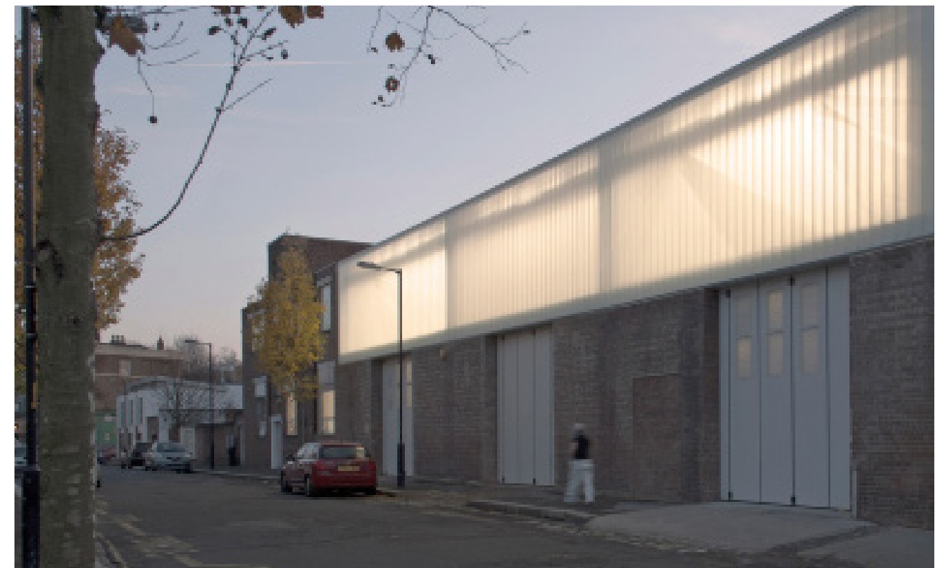
Masonry ground floor with lightweight polycarbonate cladding to first floor
