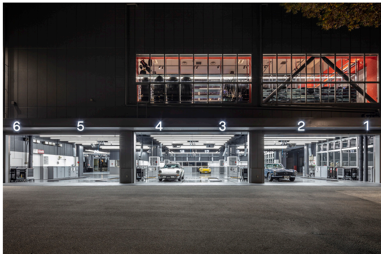
Garage/workshop with large bay openings and mezzannine level above
