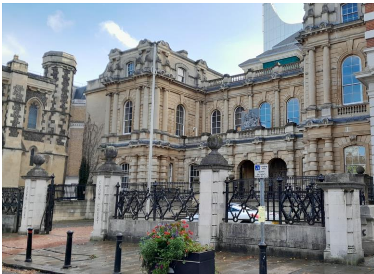
Fig 1. Old Shire Hall. Site photo taken by Case Officer on 26/10/2022
