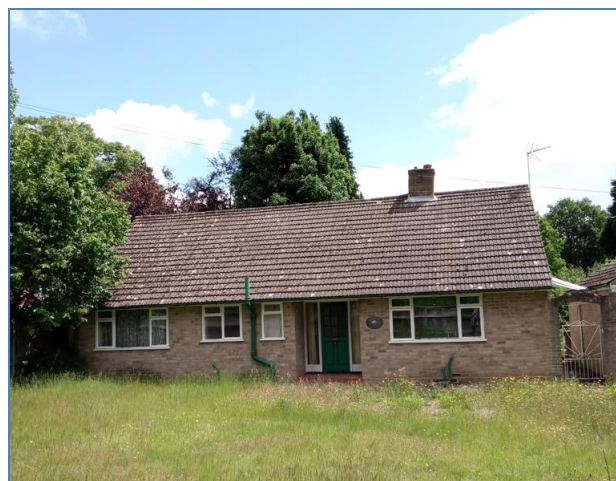
Fig 2. Existing front elevation. Site photo taken on 30/05/2022.
