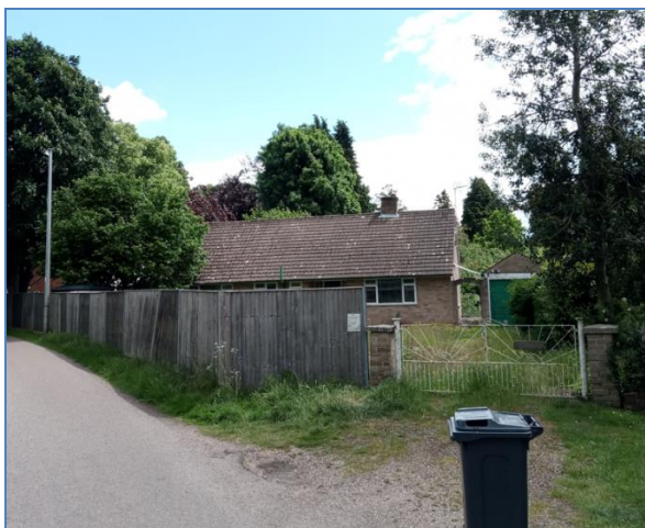
Fig 1. Existing front elevation. Site photo taken on 30/05/2022.
