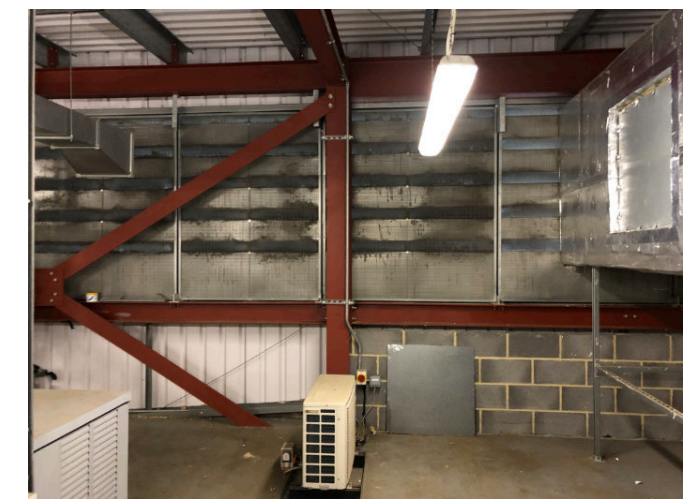
First Floor Plant Room
