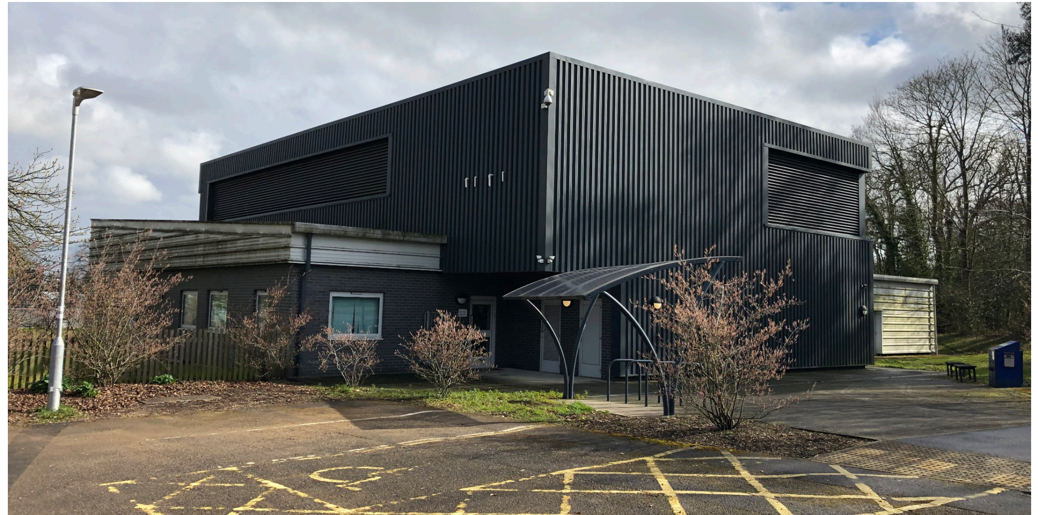
Entrance to Existing Building
