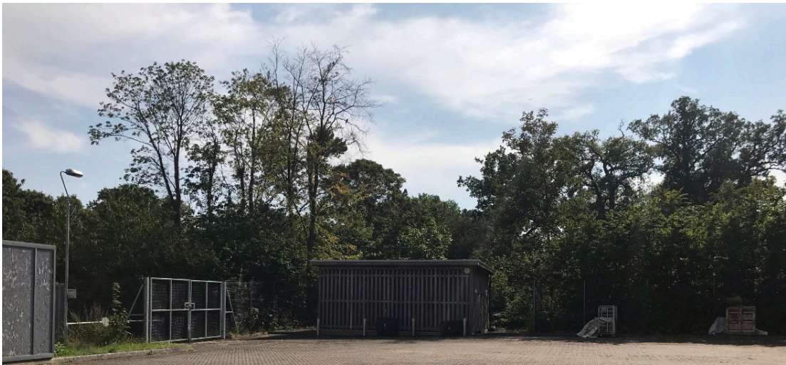
View across service yard towards substation
