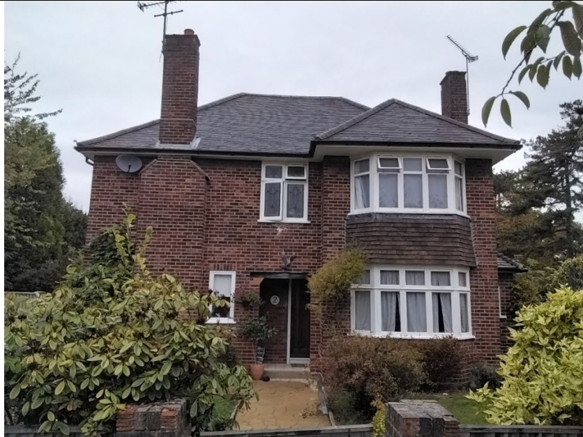
Principle elevation view from Courtenay Drive
