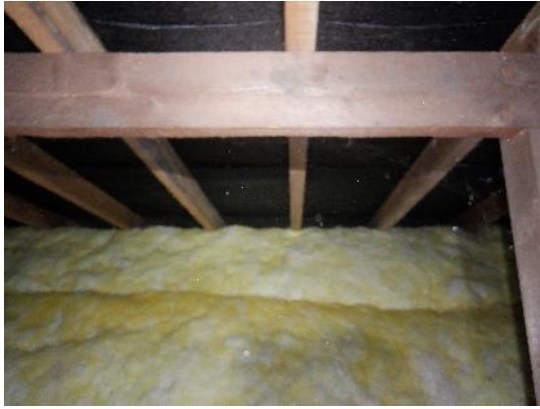
13. Fibreglass insulation along the sides of the void, up to the open eaves.
