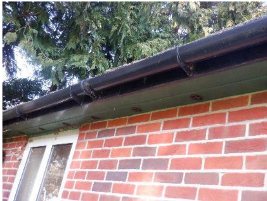
9. Flush soffit to brickwork (rear elevation).
