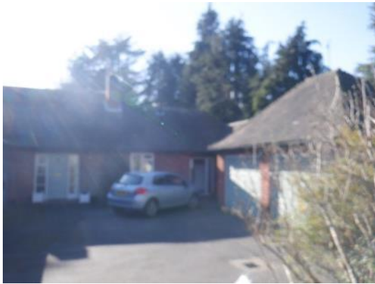
1. Front of the bungalow viewed from the east.
