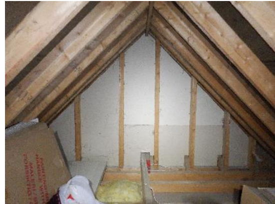
16. Plasterboard gable at the north-eastern corner of the void.
