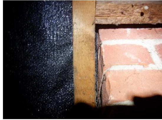
14. Roofing felt tight to brickwork chimney.
