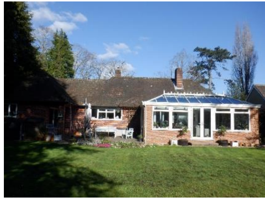
2. Rear of the bungalow viewed from the west.
