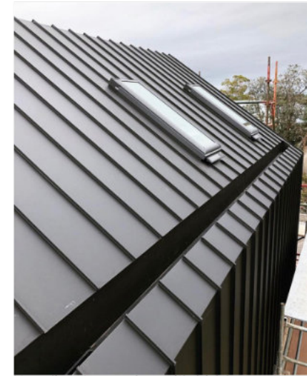
Standing Seam Zinc with hidden gutter
