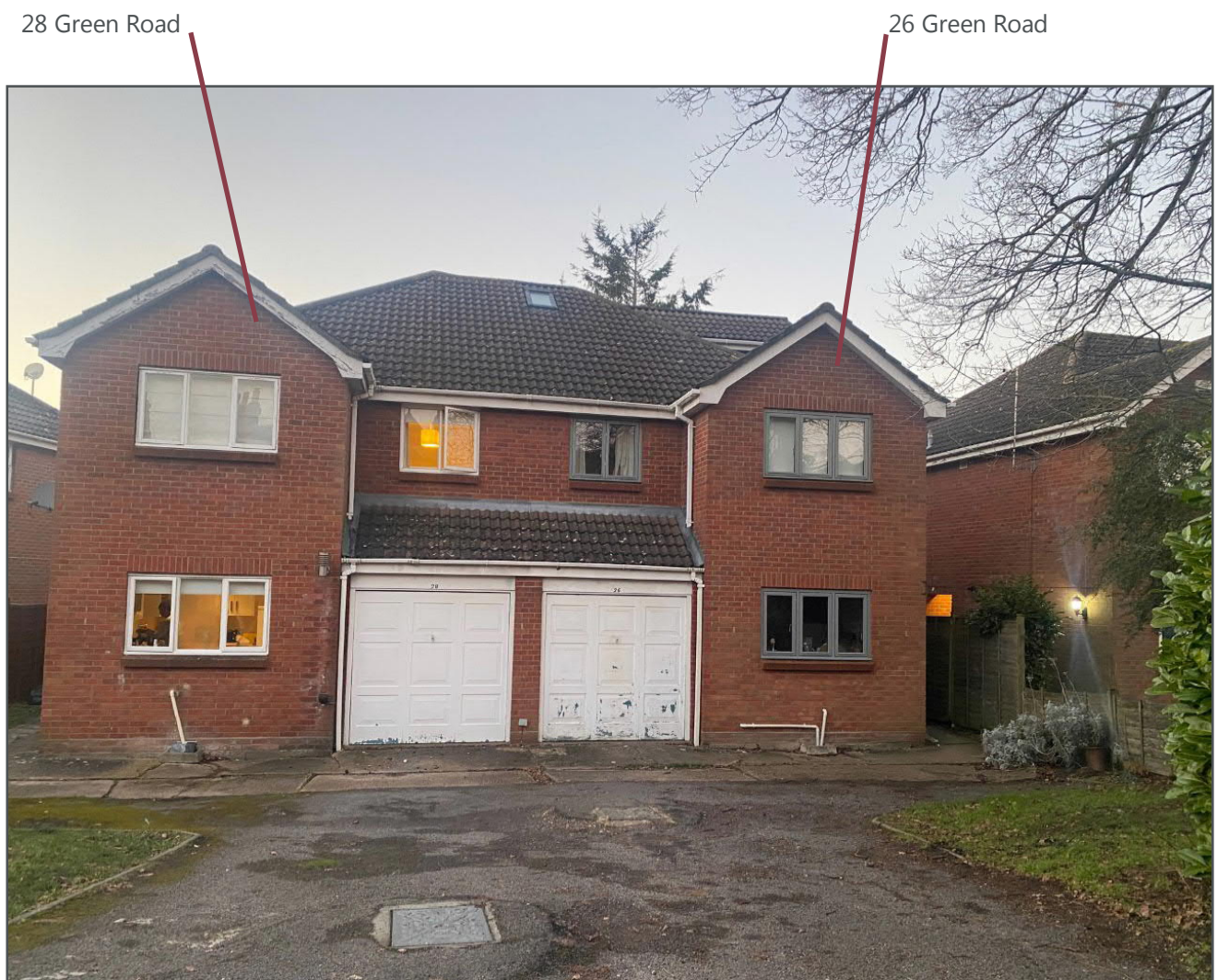
Image 1: No.s 28 and 26 Green Road, southeast elevation
