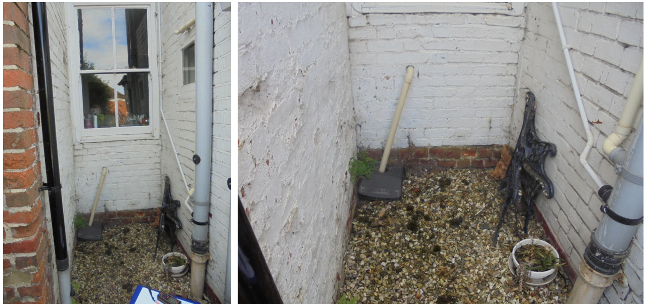
Photo 9-12 – Photos showing rear areas impacted by underpinning
