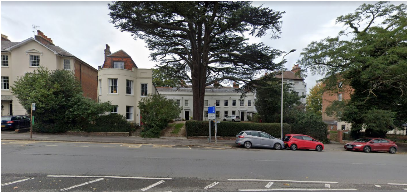
Google streetview image of the front elevation.
