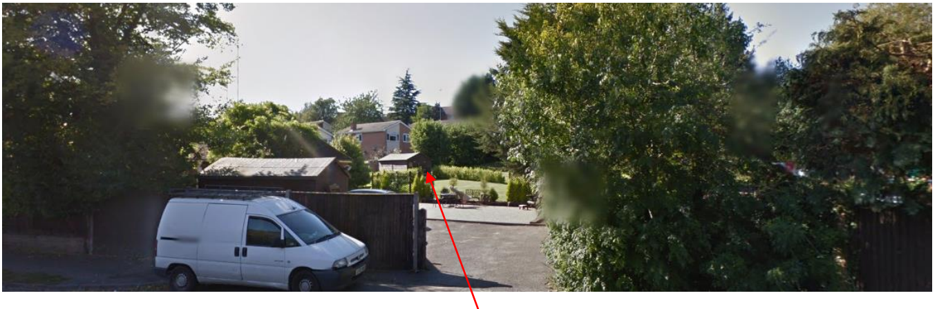
Cabin the mobile home will retrieve electricity from
