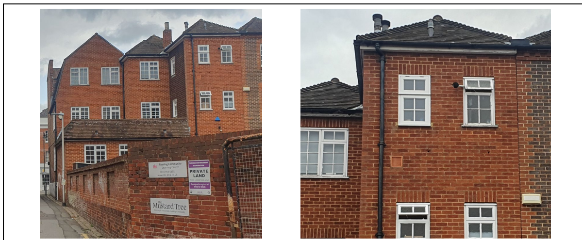
Figure 2: Site Location Measurement Pictures
