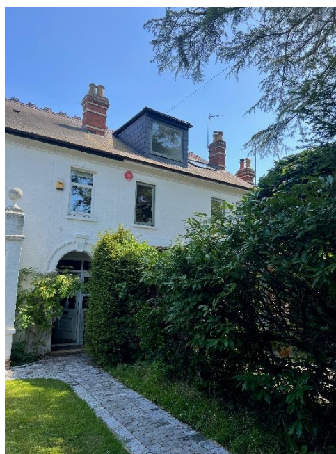
Front roof dormer projection can also be seen at neighbouring property (No. 46) Priest Hill.
