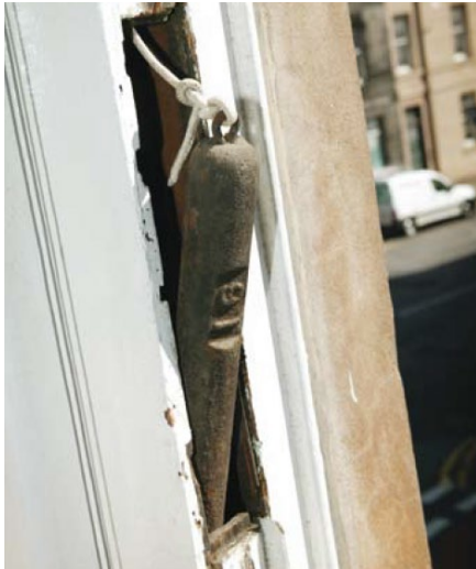
Figure 6. Access pocket to weights (Source: Historic Scotland)
