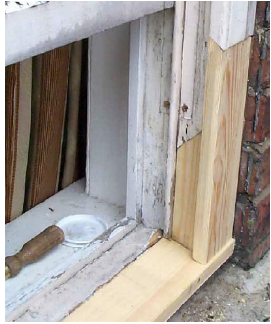
Figure 2. Half cill replacement, outer lining replaced, and part of the pulley lining replaced with new timber splices (Source: Historic England)
