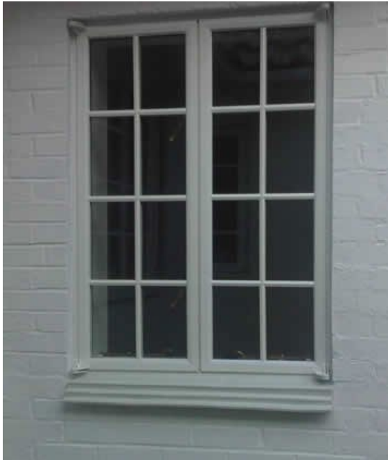
Figure 10. Thermally Broken Steel Window, achieves near identical sightlines to original Crittall windows (Source: Met therm Website)
