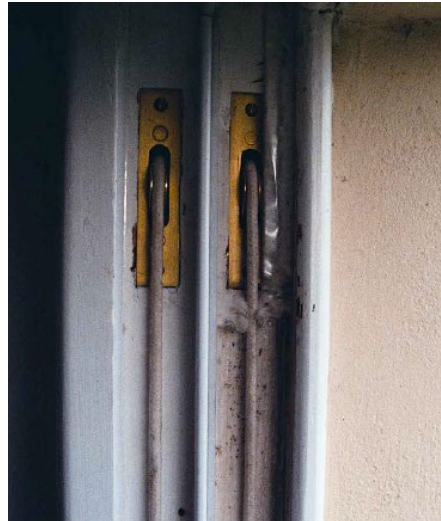
Figure 7. Brass Pulleys and Sash Cords. (Source: Historic England)
