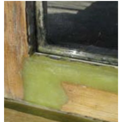
Figure 5. Resin Repair Ready to Paint. (Source: Repair Care International)
