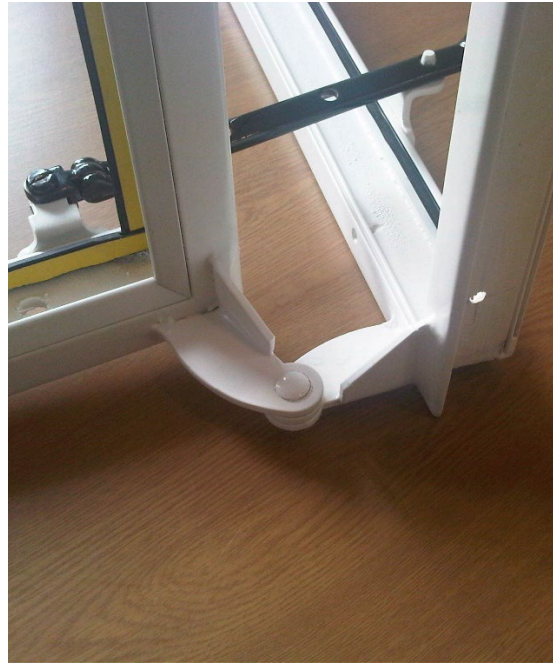
Figure 11. Projecting hinges and original ironmongery can be replicated. (Source: Met therm Website)
