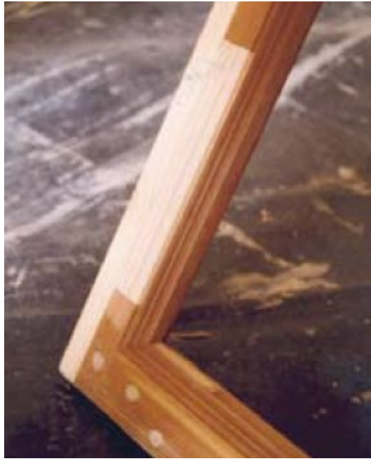
Figure 1. Joint of a sash rail and stile repaired with a timber splice, screwed and plugged. (Source: Historic Scotland)
