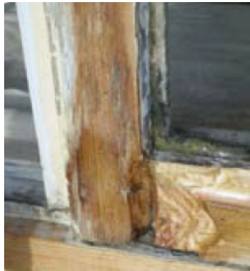
Figure 4. Sound timber primed to receive resin repair. (Source: Repair Care International)
