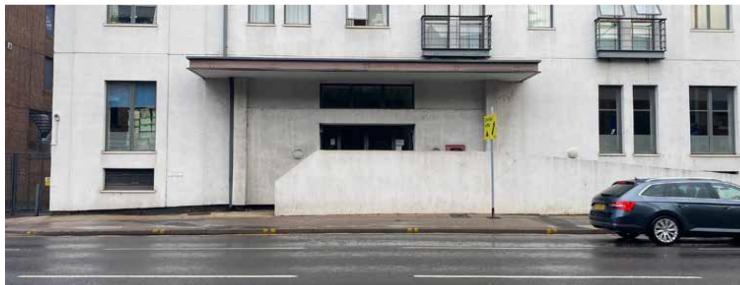
Fig. 7 Principal entrance to the office block
