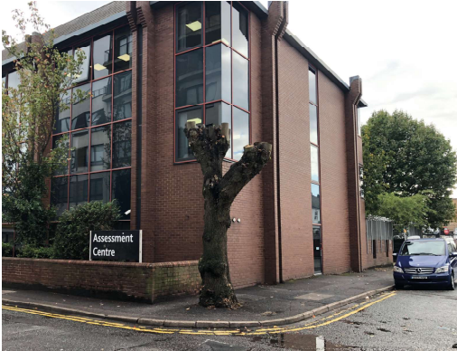
4. Corner of Eaton Place
