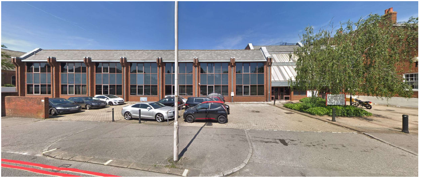
Existing Building - frontage onto Oxford Road
