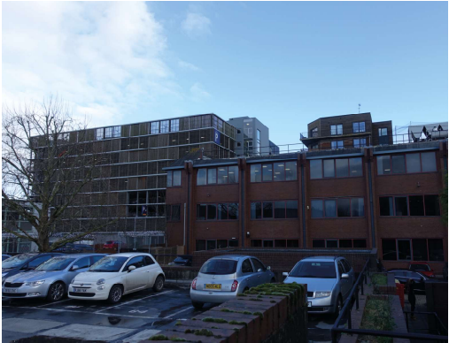
3. View from car park looking East
