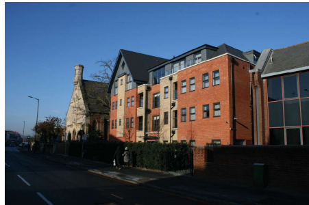
2. 114-116 Oxford Road - Looking North on Oxford Road
