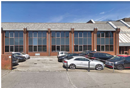
1. South Facade and existing car park - Looking from Oxford Road
