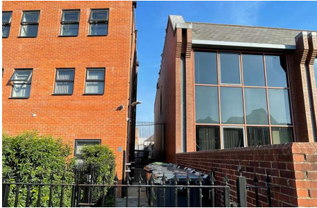
5. Windows of 114-116 Oxford Road facing towards the West Facade of Eaton Court
