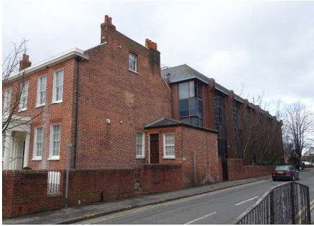
7. East Facade - Looking from Eaton Place
