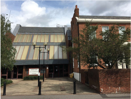
1. Junction with adjacent building on Oxford Road
