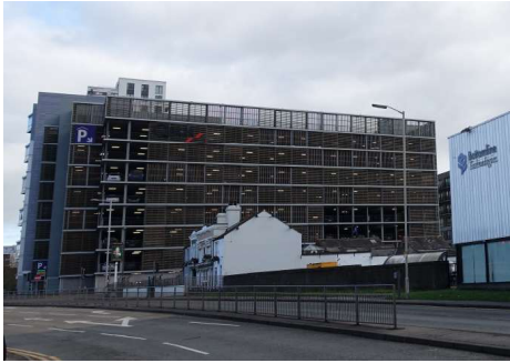
10. Chatham Place Multi-storey Carpark (9 Storeys)
