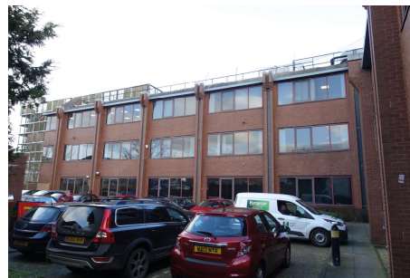
4. Eaton Court West Facade looking from car park
