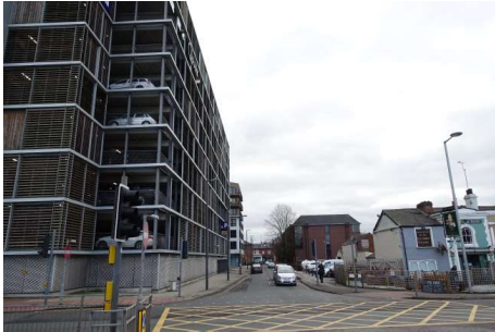
9. Looking South from Chatham Street
