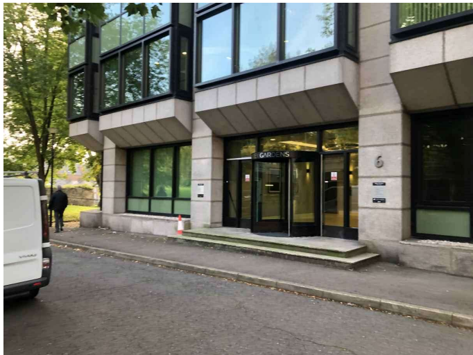
ABBEY GARDENS NORTH BLOCK – EXTERIOR - 07/10/22
