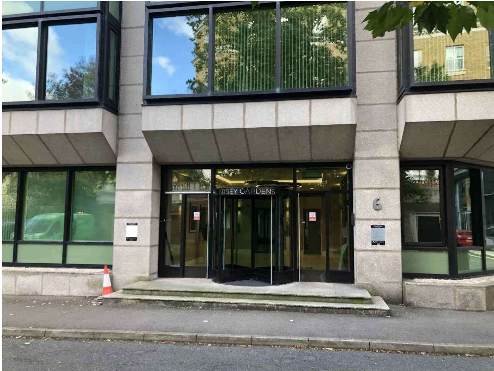
ABBEY GARDENS NORTH BLOCK – EXTERIOR - 07/10/22
