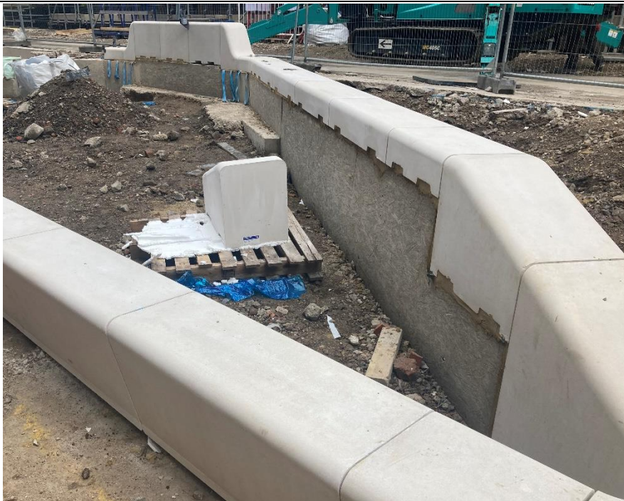
Photograph showing the condition of Area A11 during the first site visit on 8/10/2021, looking southwards. The concreting and stonework around the edges of these areas had not been fully completed, with the interiors containing Made Ground and various construction materials.
