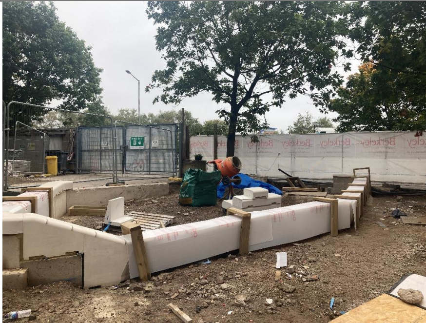
Photograph showing the condition of Area A10 during the first site visit on 8/10/2021, looking northwards. The concreting and stonework around the edges of these areas had not been fully completed, with the interiors containing Made Ground, various construction materials, and a portable cement mixer.
