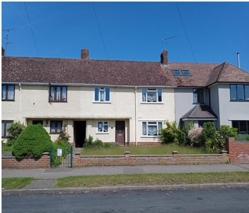
Figure 1: Existing front elevation (site visit - 27 th May 2022).
