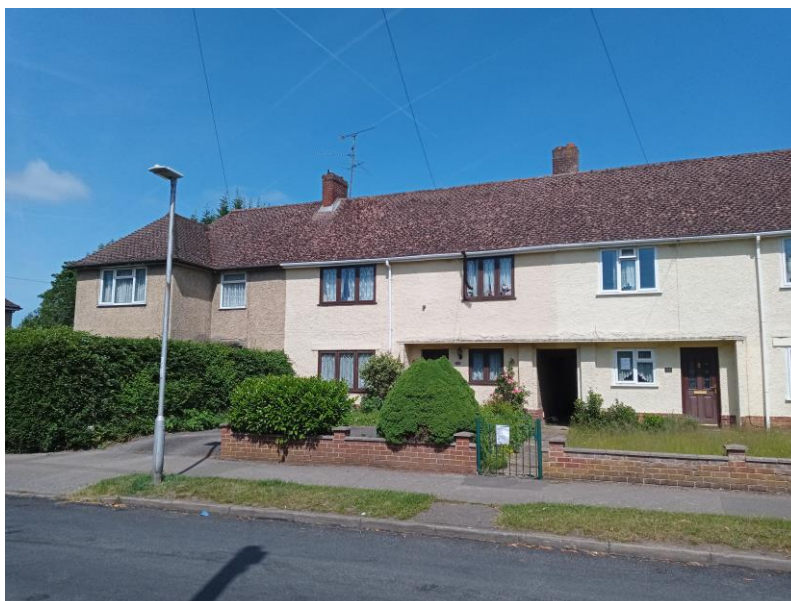
Figure 3: Existing terrace frontage (ii)
