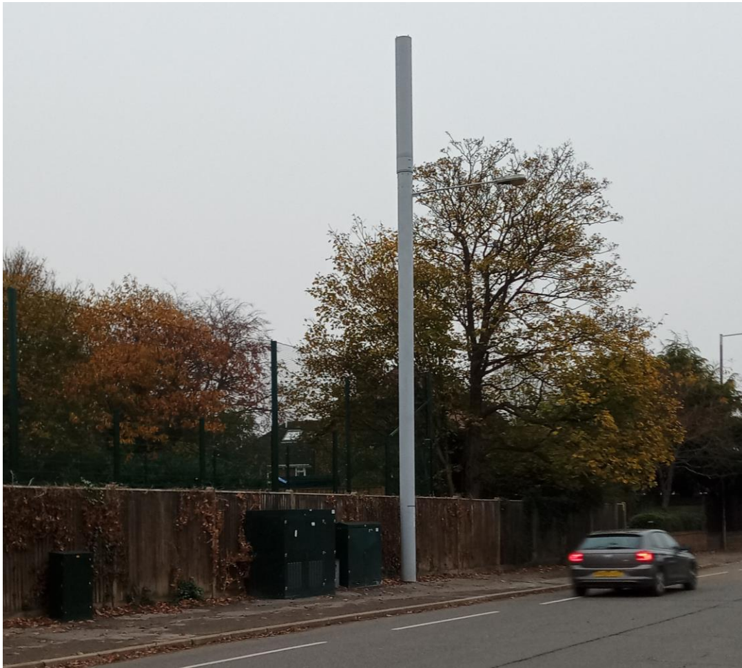
Figure 5: Existing mast approximately 80m east of the site.
