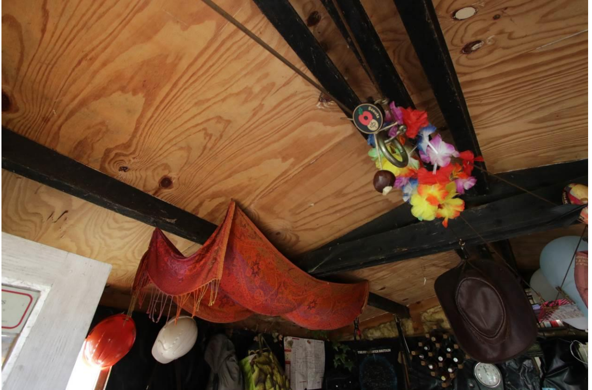
Photo 13: Roof of standalone shed. Wood with roofing felt and negligible potential for roosting features.
