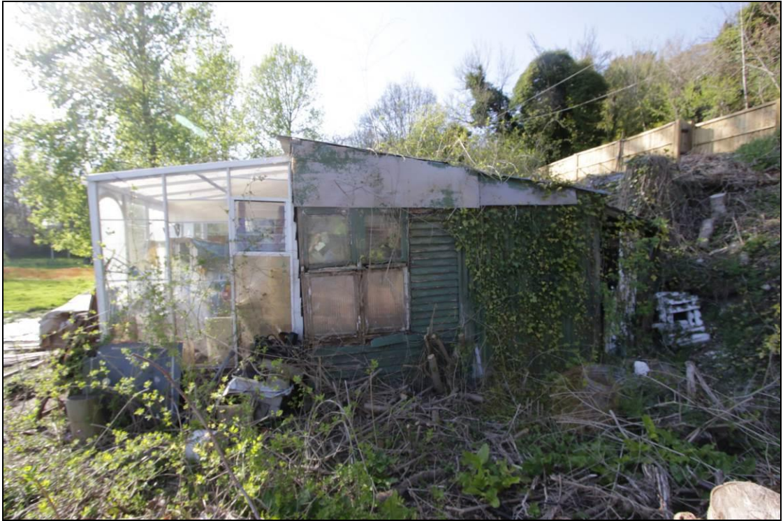
Photo 3: Shed on site with greenhouse attached, and in poor repair in places
