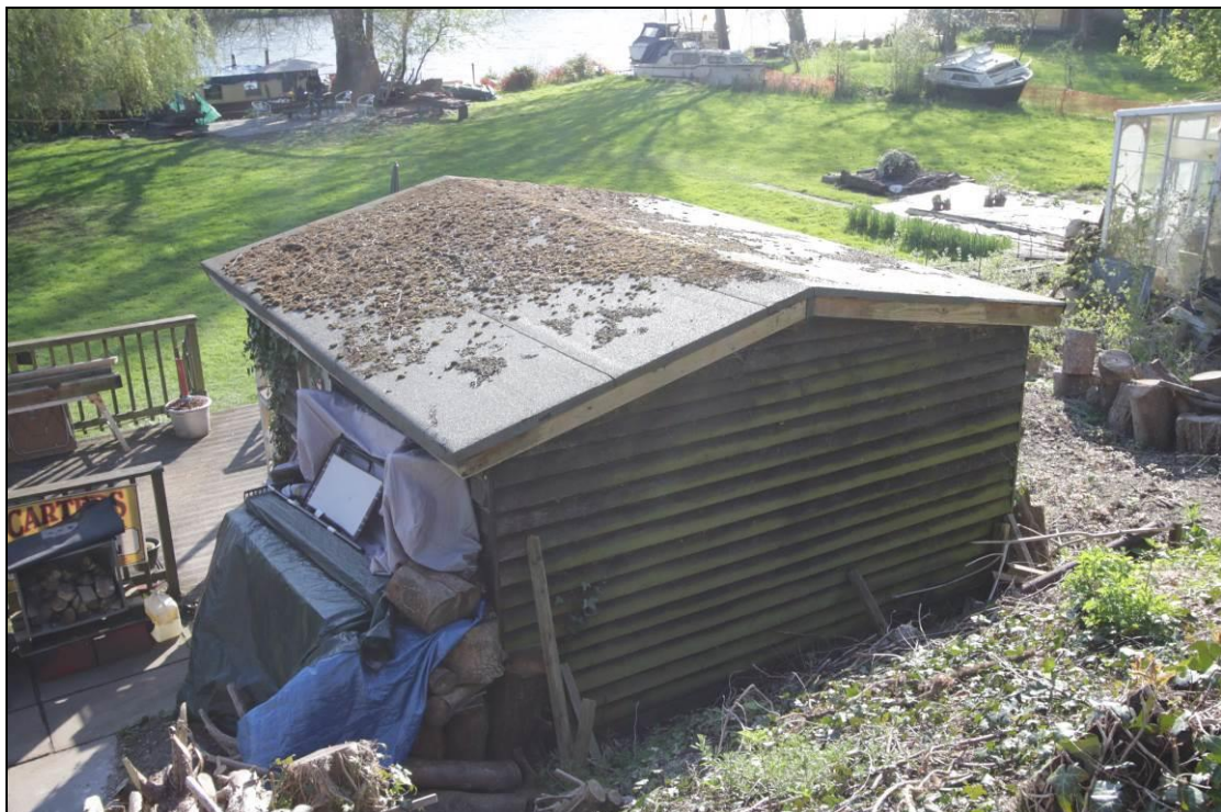
Photo 2: Shed on Site – freestanding with wooden clad sides and wood roof with felt
