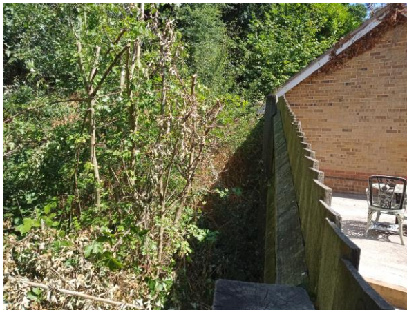
Fig 1: Existing vegetation off site (site visit 9/8/22)
